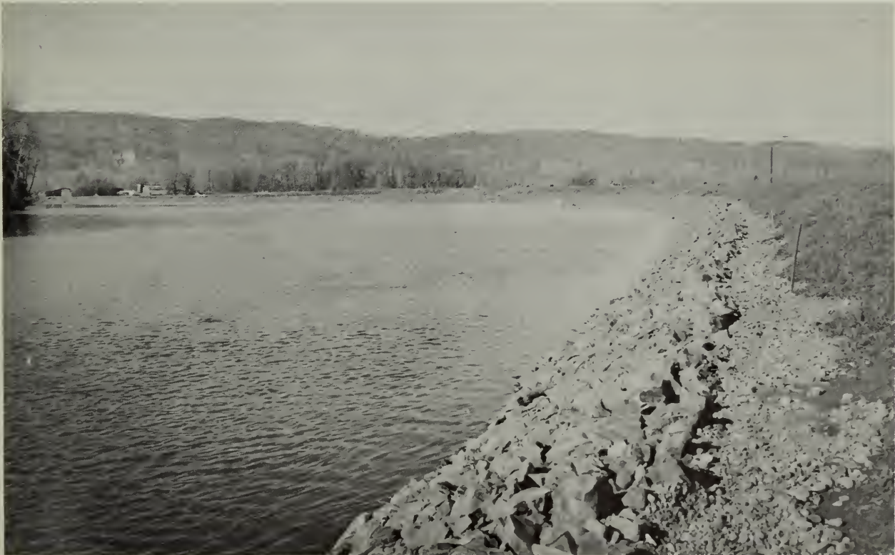
Photo 29.--This portion of the Clatskanie River bank has been protected by rock riprap, Oregon, 1962. SCS photo
