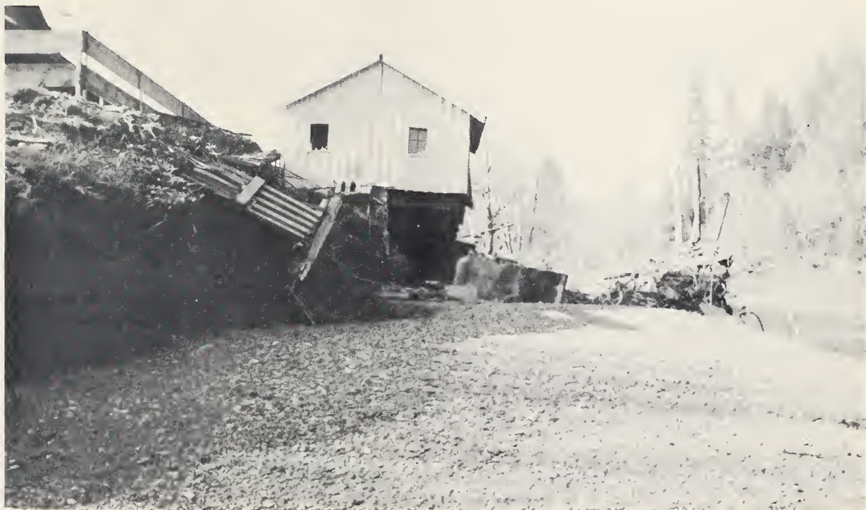
Figure 31 Riverbank erosion undercutting farm buildings and fences, Sixes River, Sixes Sub-basin, Oreg.
