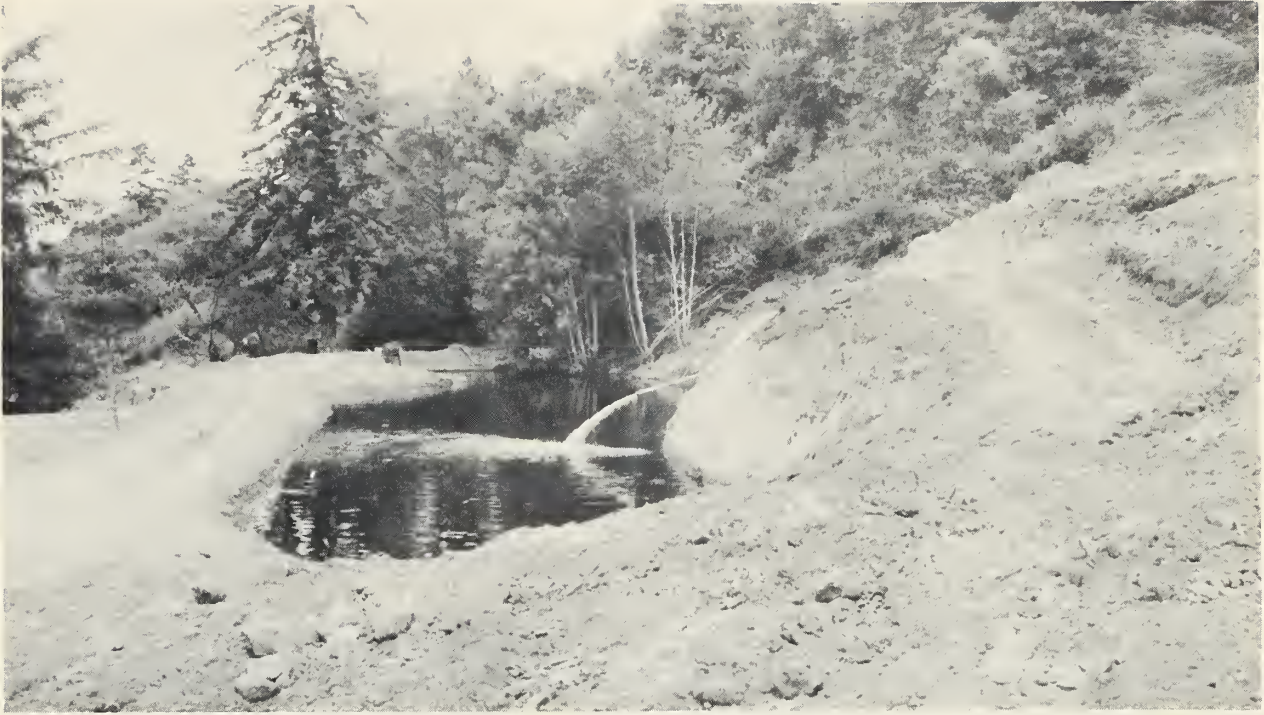
Figure 32 Overnight holding reservoir for irrigation where water supply is limited in the harbor area, Chetco Subbasin, Oreg.
