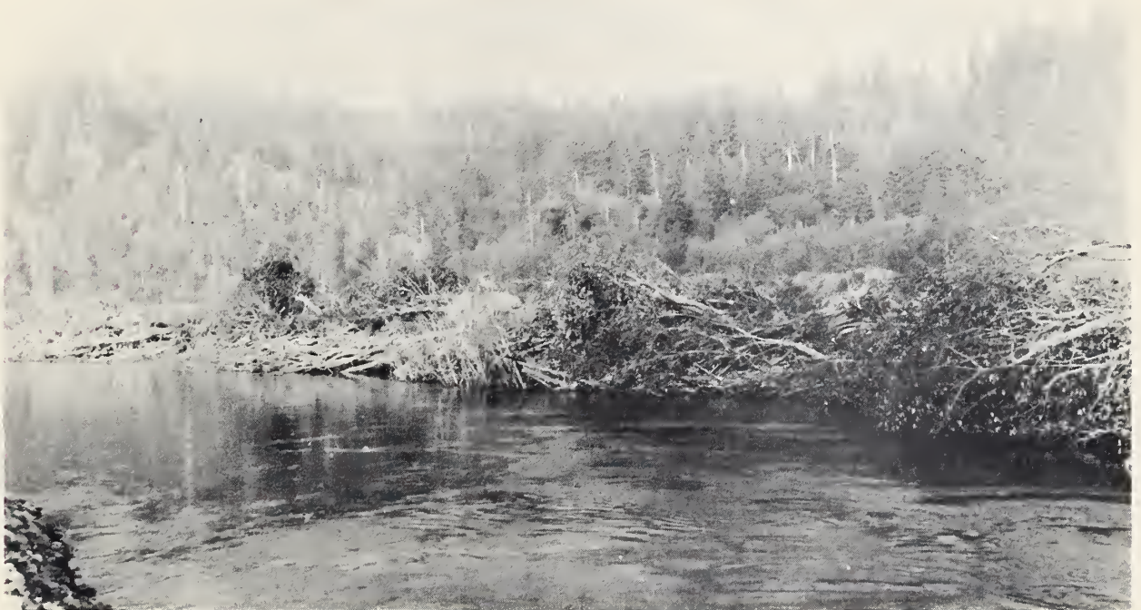
Figure 34 Myrtle trees anchored to the Sixes River bank for bank protection, Sixes Subbasin, Oreg.
