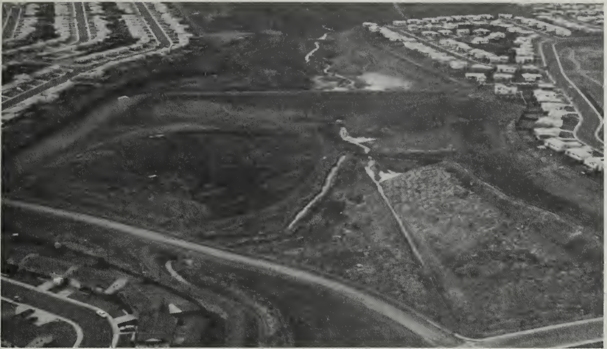
This completed PL-566 flood water detention structure is one of three such structures constructed for the Peavine Watershed Project near Reno
