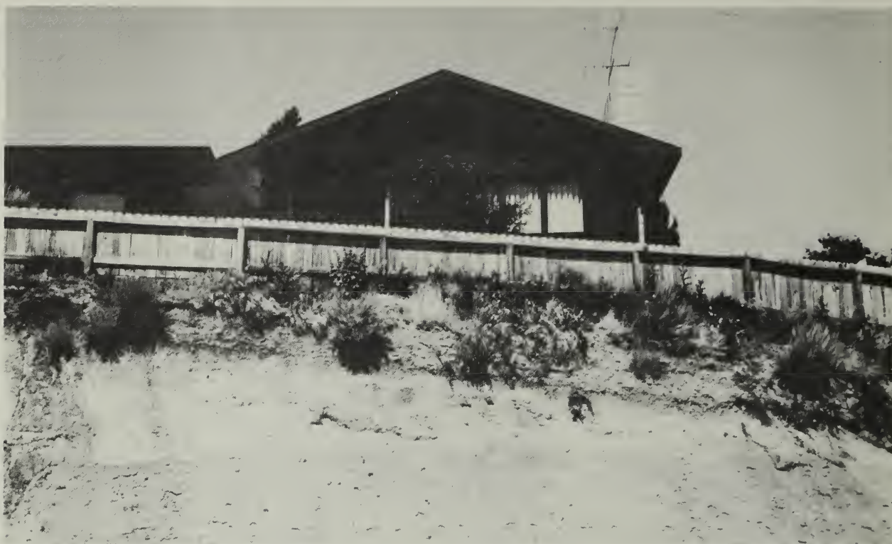
Southwest Reno. General Soil Map unit 30. Physical Land Use Suitability: grazing, rating good. Steep embankment is cut into soft bedrock creating erosion problem.
