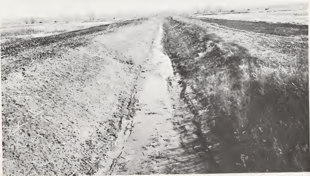
Channel Improvements are Often required in Flood-Prevention Projects
