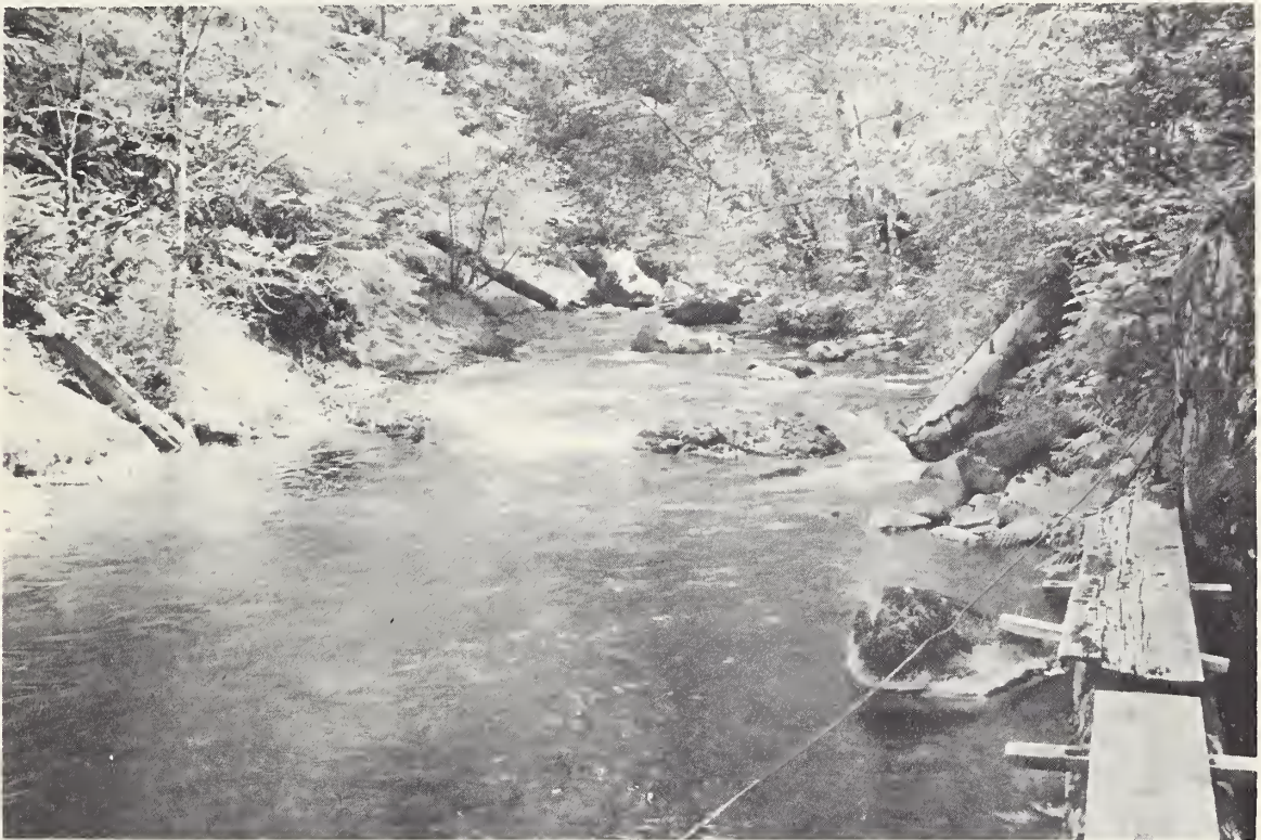
Photo 13.--South Fork Clackamas River near the Oregon City-West Linn water supply intake structure. FS photo. NO. 485520
