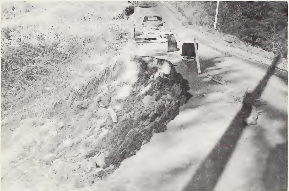
Photo 23.--A road slide is the result of heavy and prolonged rains and floodwaters, subbasin 8. SCS photo. 7-597-11
