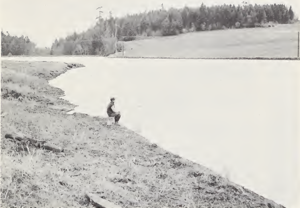
Photo 36.--A typical medium sized reservoir constructed for multiple use in subbasin 8. SCS photo. 7-616-12
