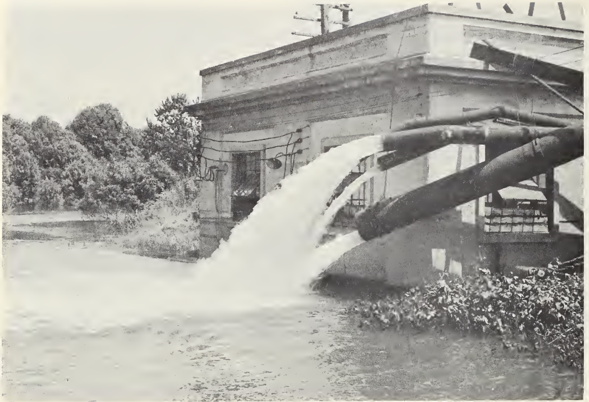
Photo 21.--Five extra pumps were placed and operated in addition to the permanent ones in the Scappoose Drainage District to keep up with the increased seepage from the 1948 flood on the Columbia River. SCS photo. 8-300-1
