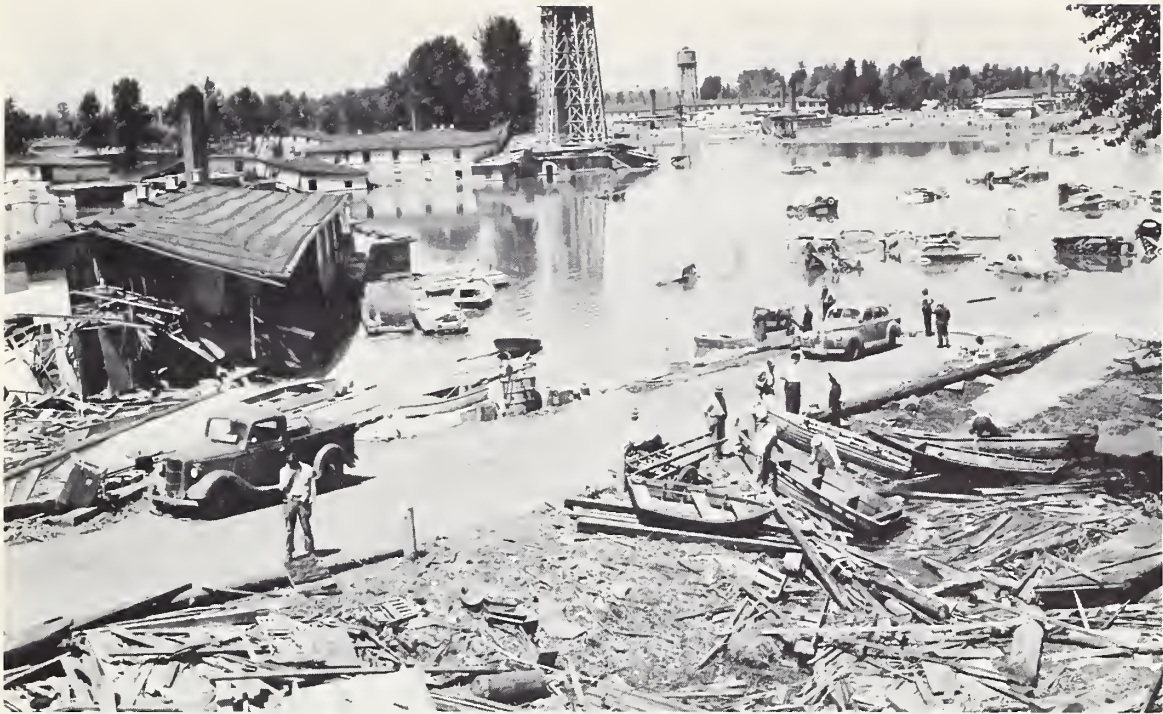
Photo 19.--This is all that remained of Vanport, Oreg., following the 1948 Columbia River flood, subbasin 10. SCS photo.
