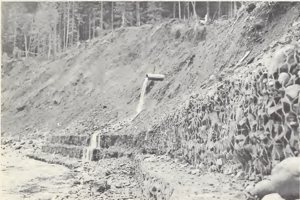
Photo 26.--A creek bank and rural road protected by wire-bound rock riprap, subbasin 9. Survey Party photo. 7-1378-8
