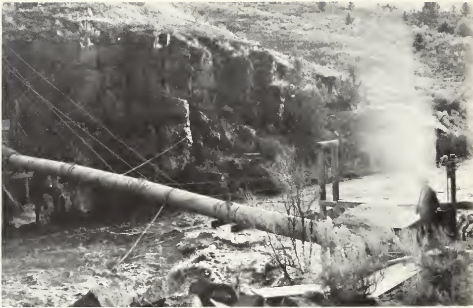
Figure 14 Irrigation structure across John Day River near Dayville, Oregon. Capacity 8 c.f.s.
