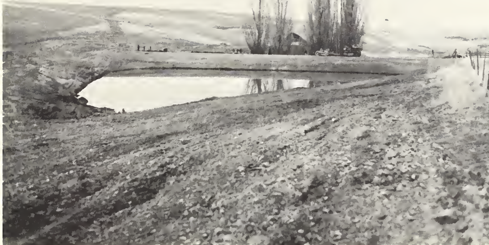
Figure 26 A typical combination earthfill and excavated stockpond nearing completion in sub-basin 3.
