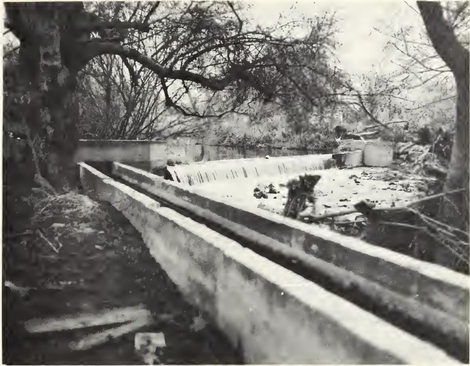
Figure 21 Concrete diversion dam with controlled flume outlet on Rock Creek, subbasin 3.
