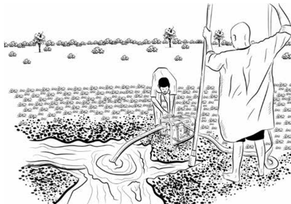
Connect pump for jetting with drilling pipe, lift water into the mud pit and ensure tight connections
