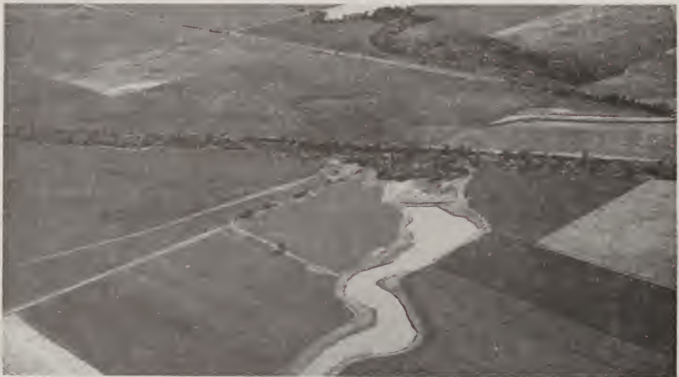
Grade Stabilization Structures Control Gullies, Reduce Erosion and Establish Base Grade for Land Treatment Measures
