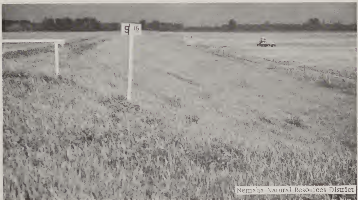
Agricultural Levee - Part of the Missouri River System
