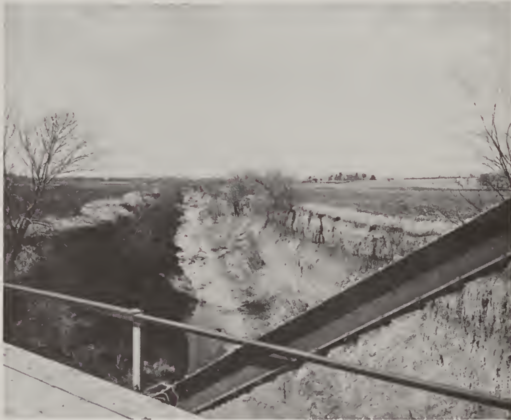
Streambank Erosion Damages Agricultural Land
