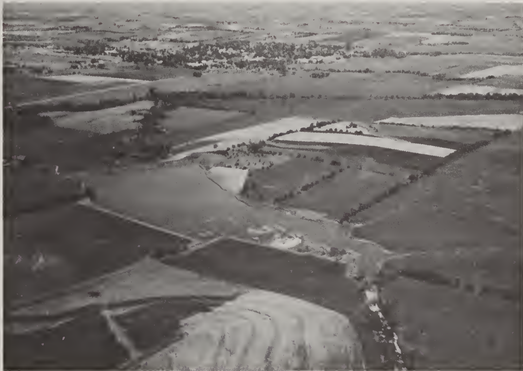
Floodwater Retarding Structures Protect Downstream Properties
