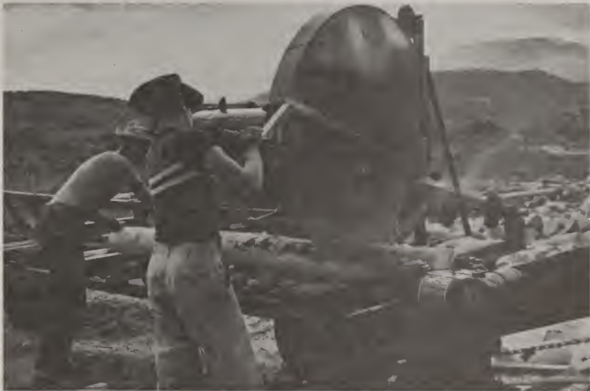
Aspen logs are cut into bolts, transported to Cedar City, and converted to excelsior.
