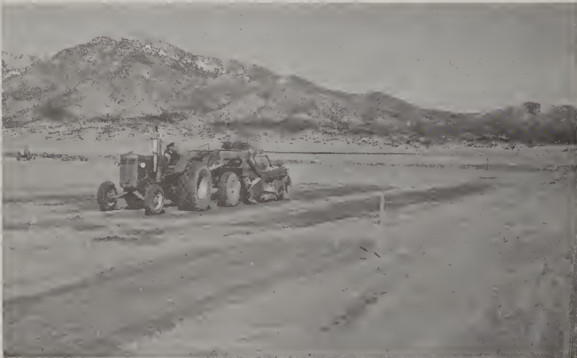
Land leveling is essential to efficient irrigation in many areas of the Basin.
