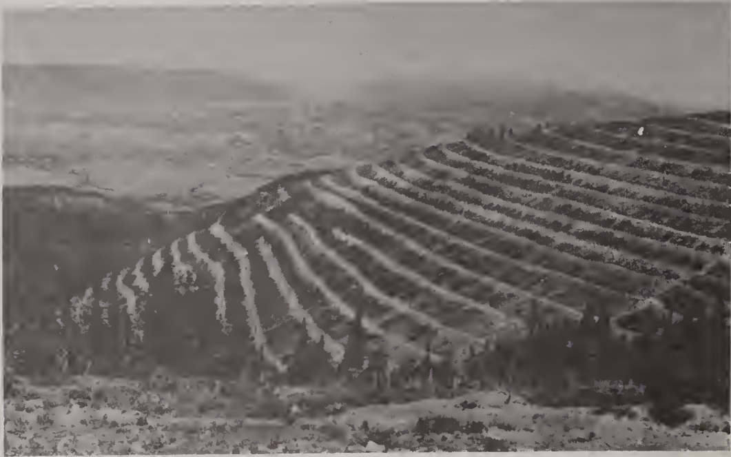
Contour trenches help stabilize a critical area at the head of Meadow Creek in the Fillmore subbasin.
