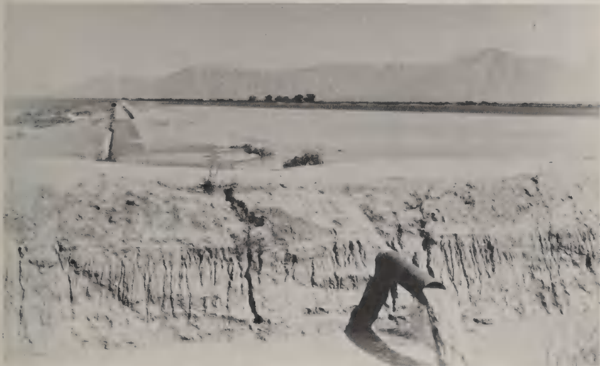
Photograph 1. A lettuce crop was completely lost when a section of dike (foreground) broke, allowing floodwater to inundate the field behind the dike. Notice flood flow damage to the ditch on the left side of the field. (SCS Photograph)
