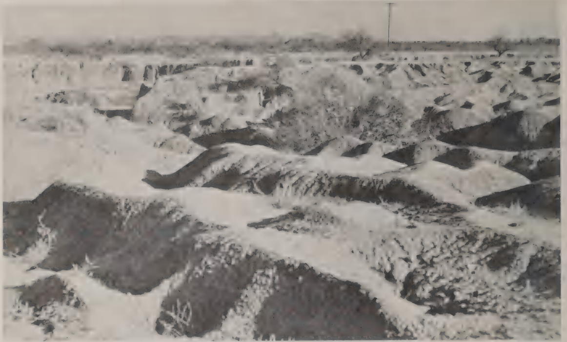
Photograph 10. Erosion class 1, erosion along San Pedro River near St. David. Areas of class 1 erosion are too small to be shown on the Erosion Classification Map. (FS Photograph)
