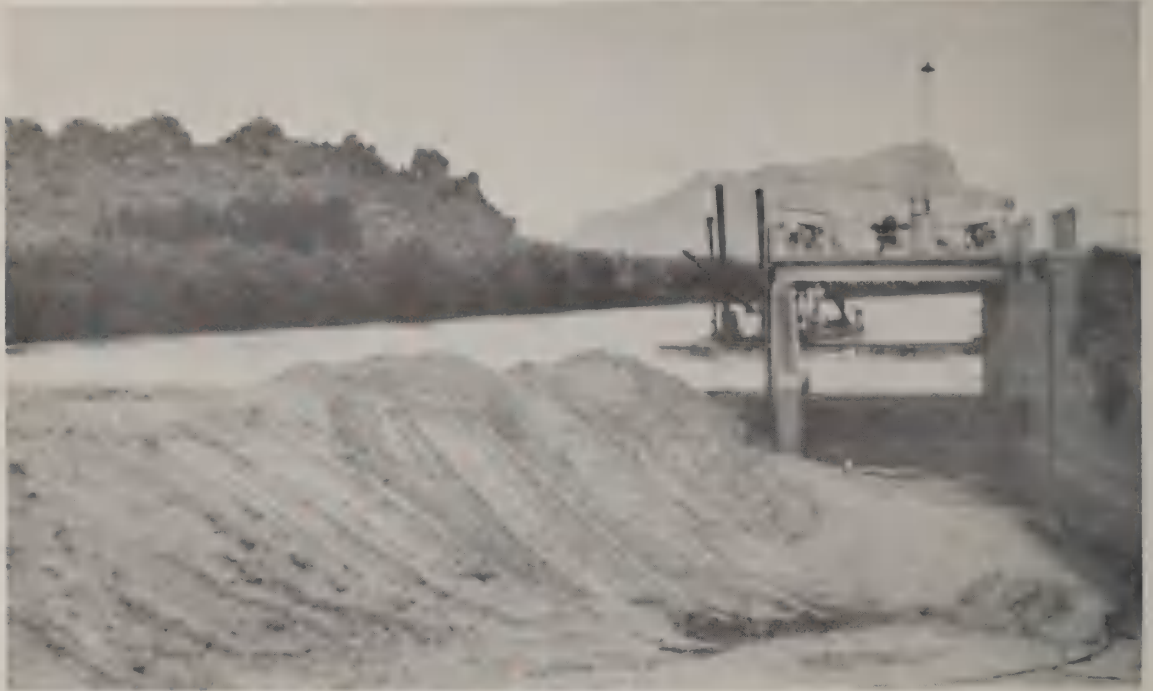
Photograph 18. Ashurst-Hayden Diversion Dam: Dredge in right background is continuously removing sediment near inlet to Florence-Casa Grande Canal. (SCS Photograph)
