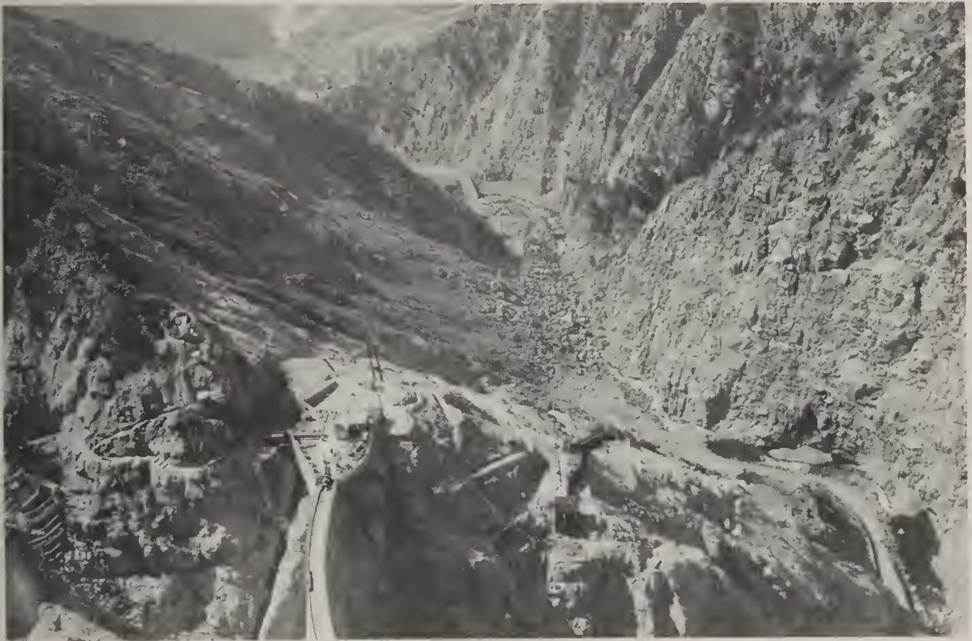
The same 1971 earthquake closed the road and inflicted about $2 million of damage to the abutments of Pacoima Dam.
