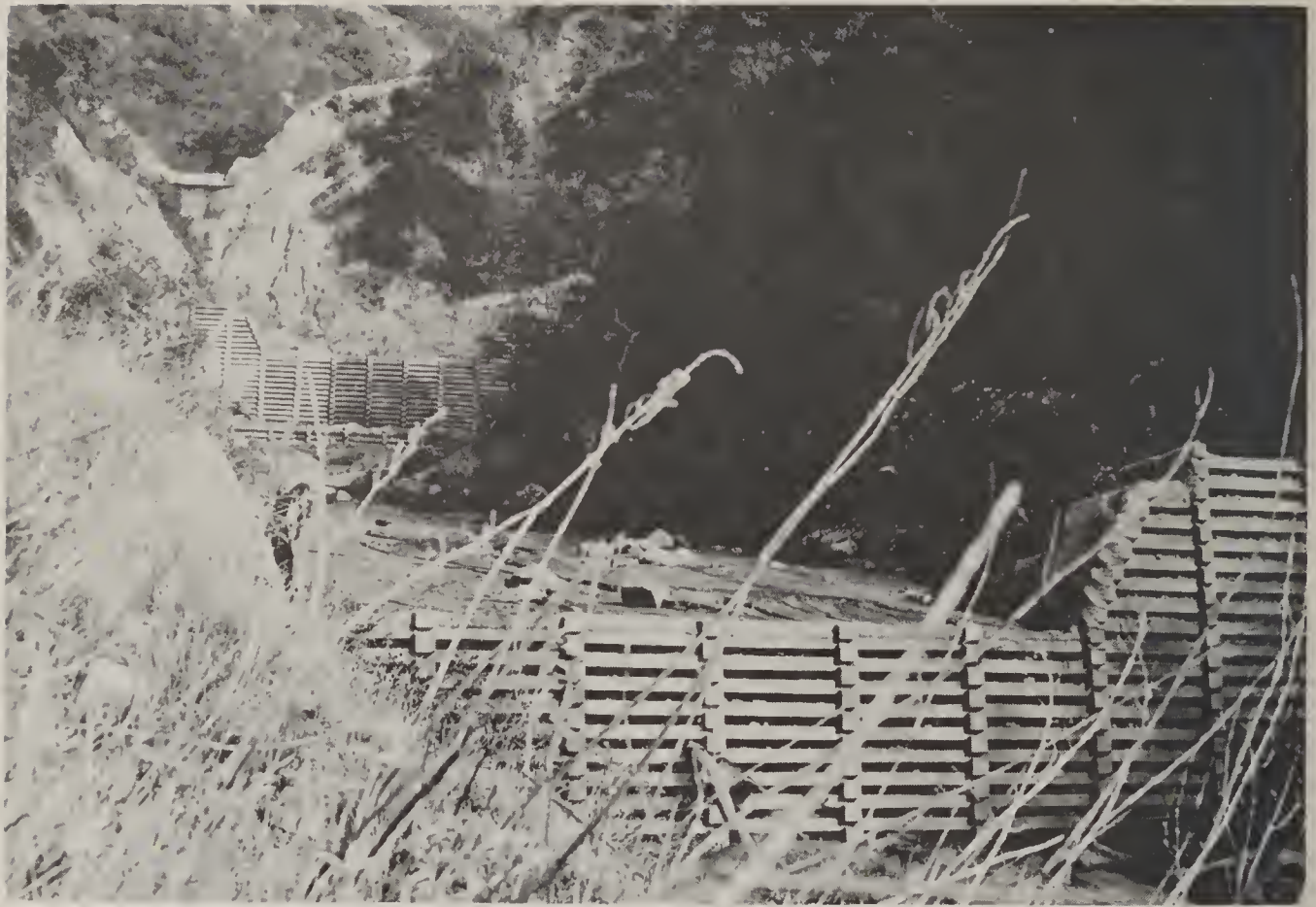
Crib structures pictured above and in diagram below are a means of stream bank stabilization and sediment storage.
