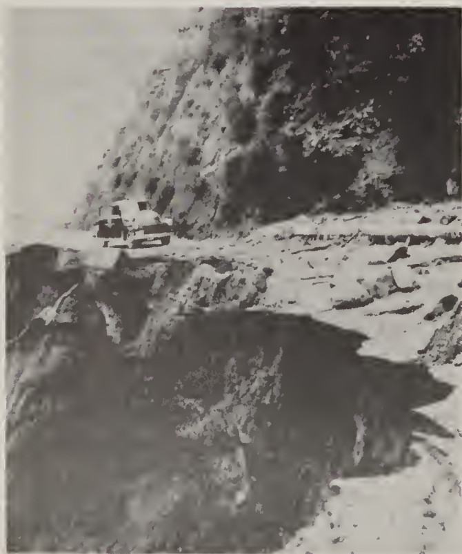
Road failure caused by flooding.
