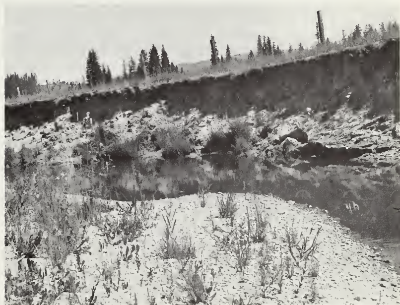
Stream Channel Erosion -- SCS Photo
