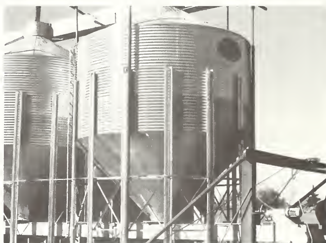
Figure 9. Bulk Storage of Cubes in Hopper Bottom Bins.
