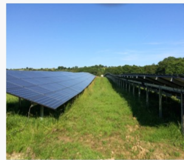
photovoltaic with restored ecosystem
