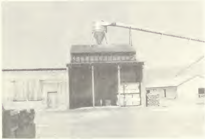
Figure 3.--Facilities used in the production of baled wood shavings.
