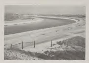
CALIFORNIA AQUEDUCT — A MAJOR CEMENT LINED CANAL USED IN TRANSPORTING WATER FROM NORTHERN CALIFORNIA.
