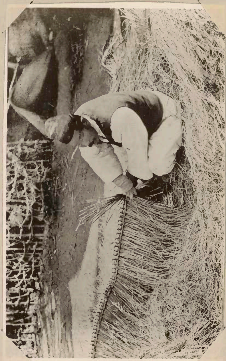
Fig. 26. Preparing rice straw for a thatched roof in Korea
