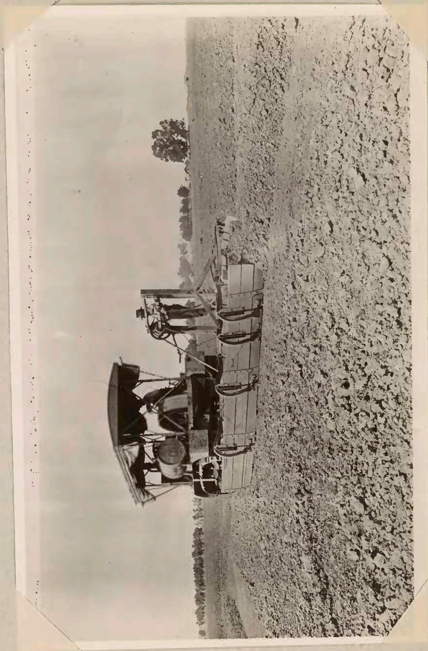
Fig. 5. Building a levee with a "checker" in California
