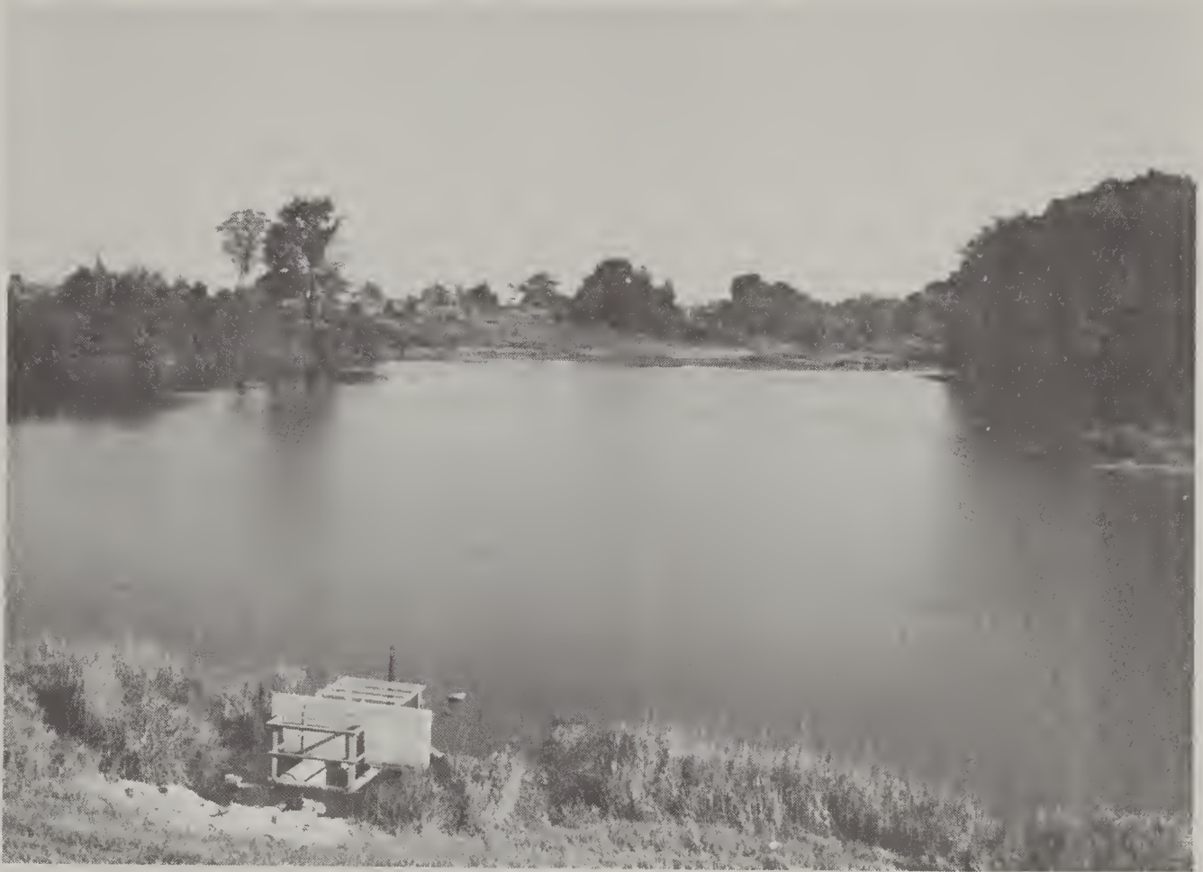
Single-purpose floodwater retarding reservoir, Chippewa Creek Watershed.
