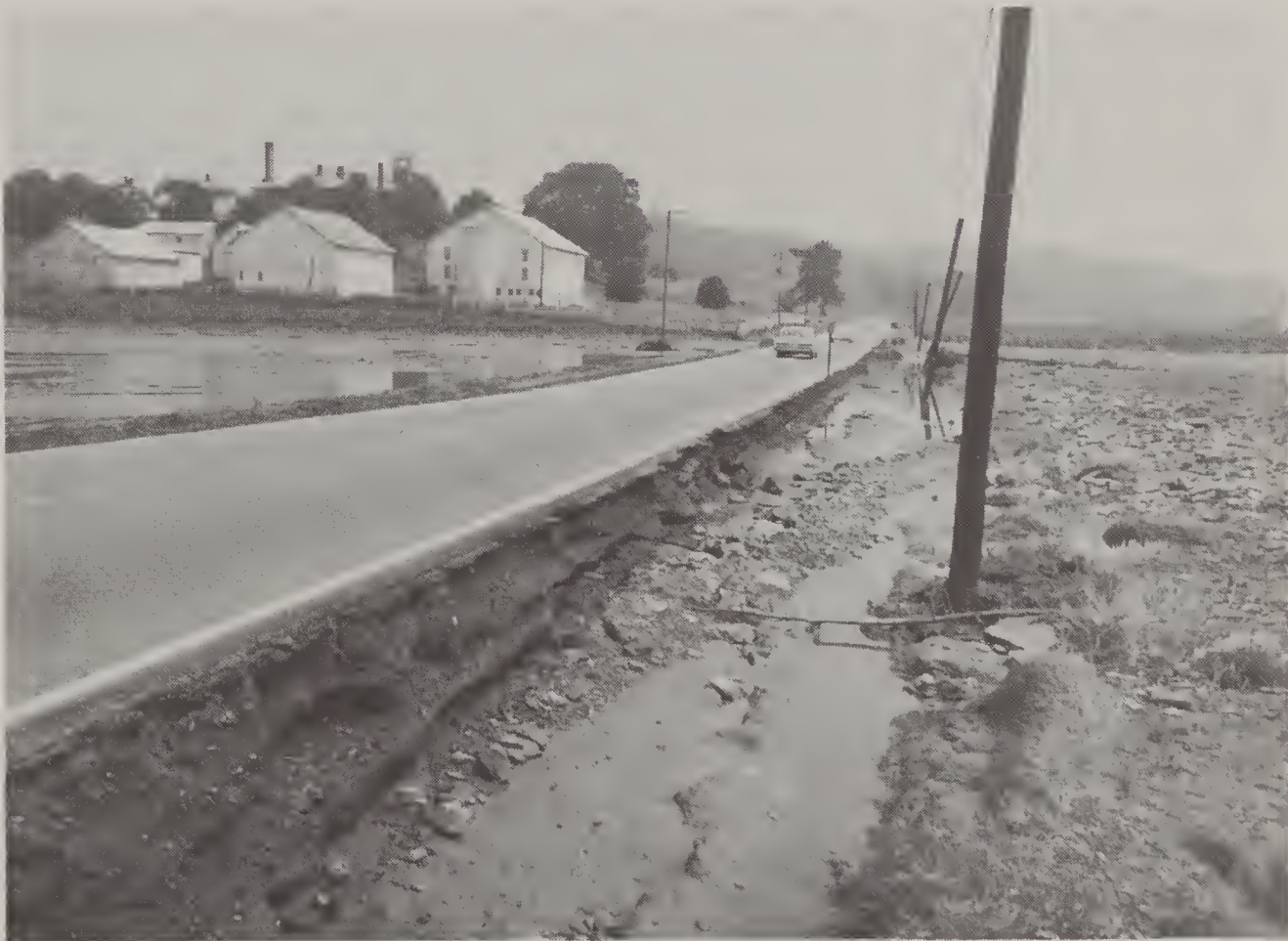
Road and bridge floodwater damage occurs throughout the basin and represents a large economic loss.
