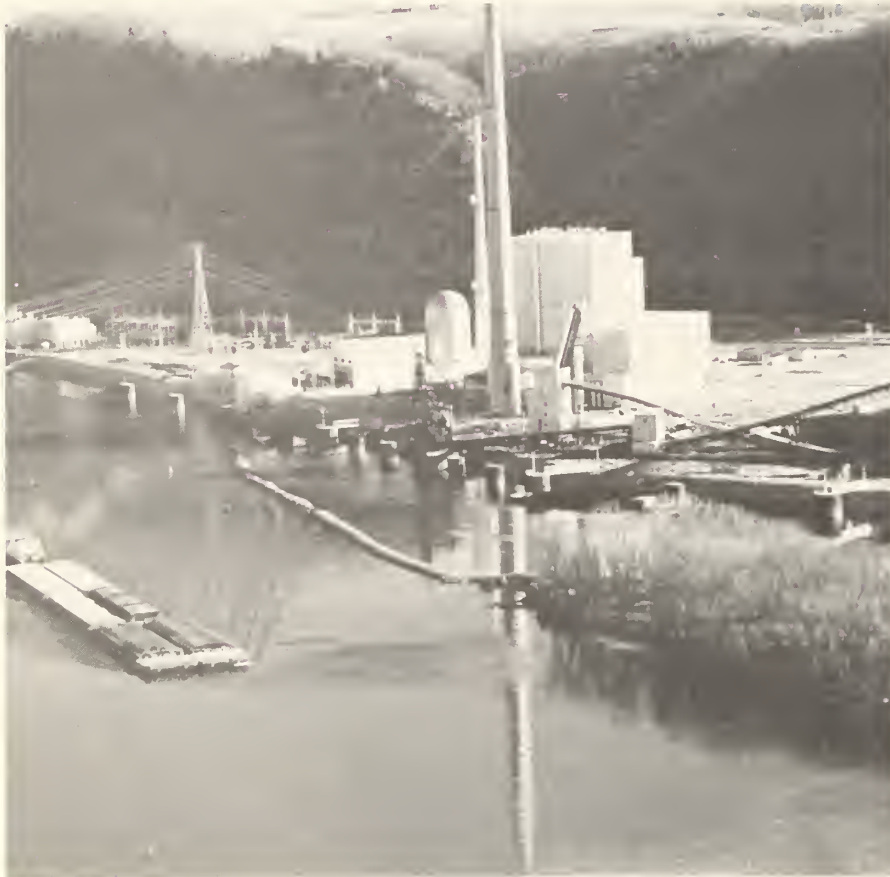
A 14,000-kilowatt generating plant built in 1941, far left, contrasts with a 300,000-kilowatt unit, center. An experimental 50,000-kilowatt nuclear plant (round dome) was completed in 1969.
