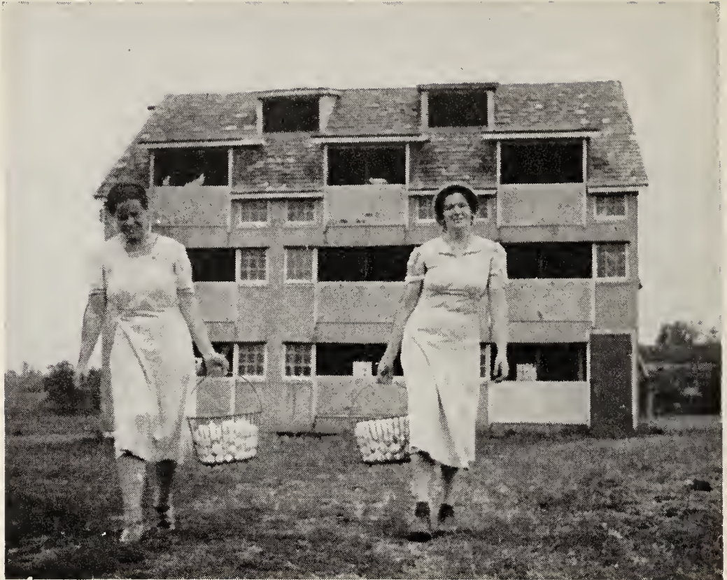
Figure 27. Installation of numerous windows and a floor in the haymow turned this barn into a good three story poultry house. (U.S.D.A.)
