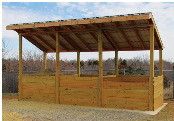
Photograph 2. A Permanent Three-Bin Wooden Mortality Composting Structure.
