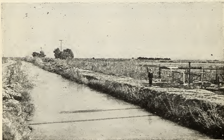
Figure 126. Most irrigated areas obtain water from rivers and creeks and by means of a diversion dam divert the water, through a ditch, to the land where it is to be used. (U. S. D. A.)
