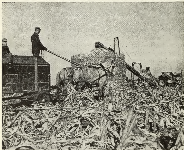
Figure 31. Corn harvesting in the Corn Belt is mostly mechanized. A mechanical picker picks the ears from the stalks and tosses them into a trailer truck. From the truck, which is hauled to the cribs by horses, or tractors, the ears are elevated mechanically to a well-ventilated crib to dry. (U. S. D. A.)
