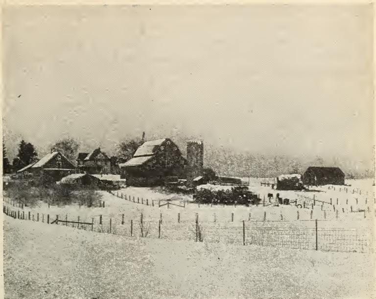
Figure 98. Good buildings on a middle western farm. (U. S. D. A.)
