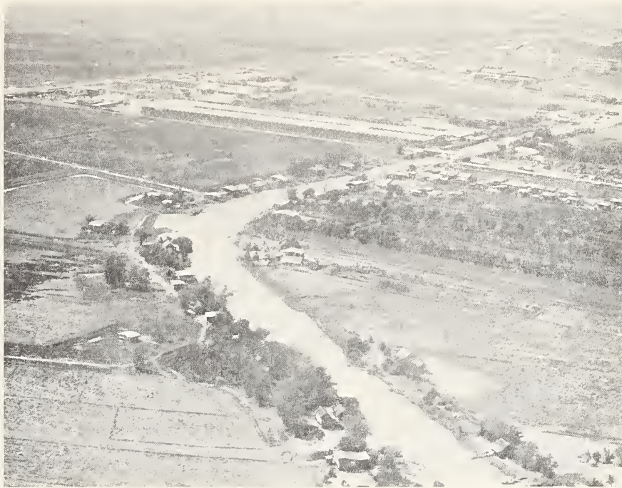
Figure 2.--Irrigation canal in Central Plain.
