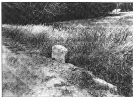
Figure 2: Concrete Headwall Partially Removed
