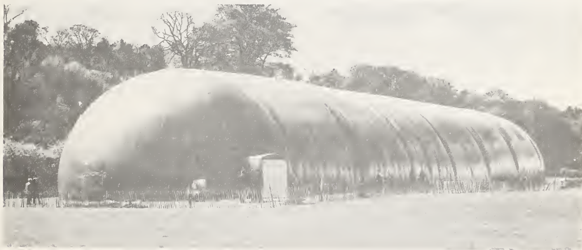
An inflated, plastic warehouse owned by Kenya's Maize and Produce Marketing Board and used for storage of corn for domestic, East African Community, and overseas markets. This portable warehouse, which can house 50,000 bags of corn, or 4,536 tons, is moisture-proof and can be fumigated.
