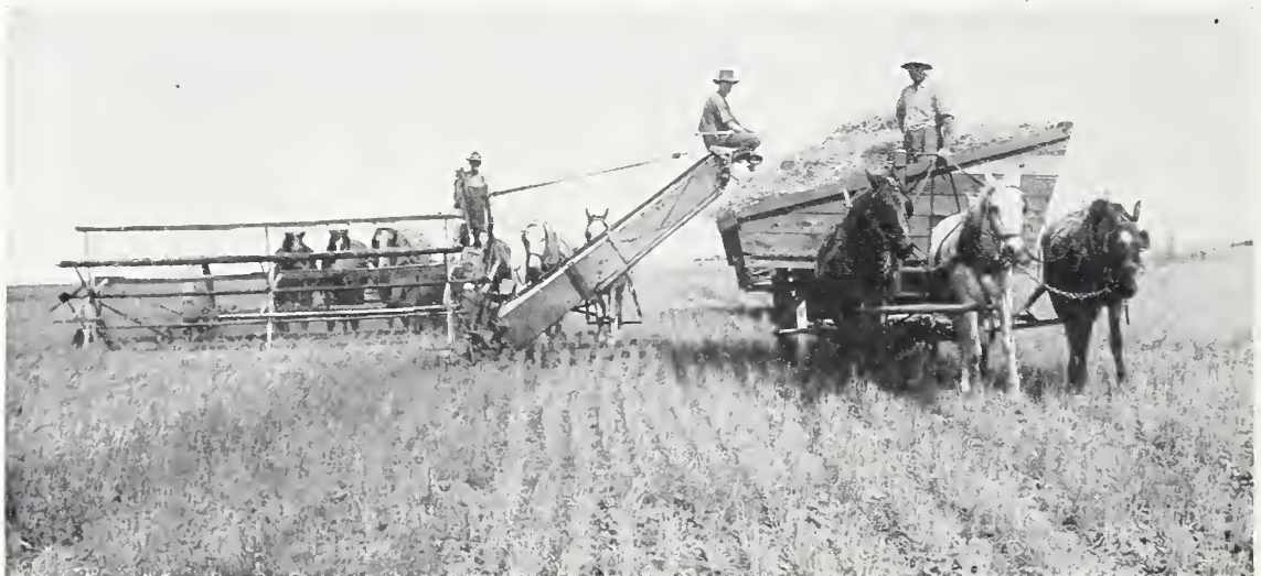
FIGURE 19.—Before the coming of the combine, the header was used extensively for harvesting small grains, especially wheat, in the subhumid parts of the Great Plains and in the Pacific Northwest. By 1920, only about 20 percent of the wheat acreage was harvested with the header, and today only about 1 percent is so harvested. A 12-foot header, with a crew of about 6 men and 12 horses, can usually cut and stack about 30 acres of 15-bushel wheat in a 10-hour day.
