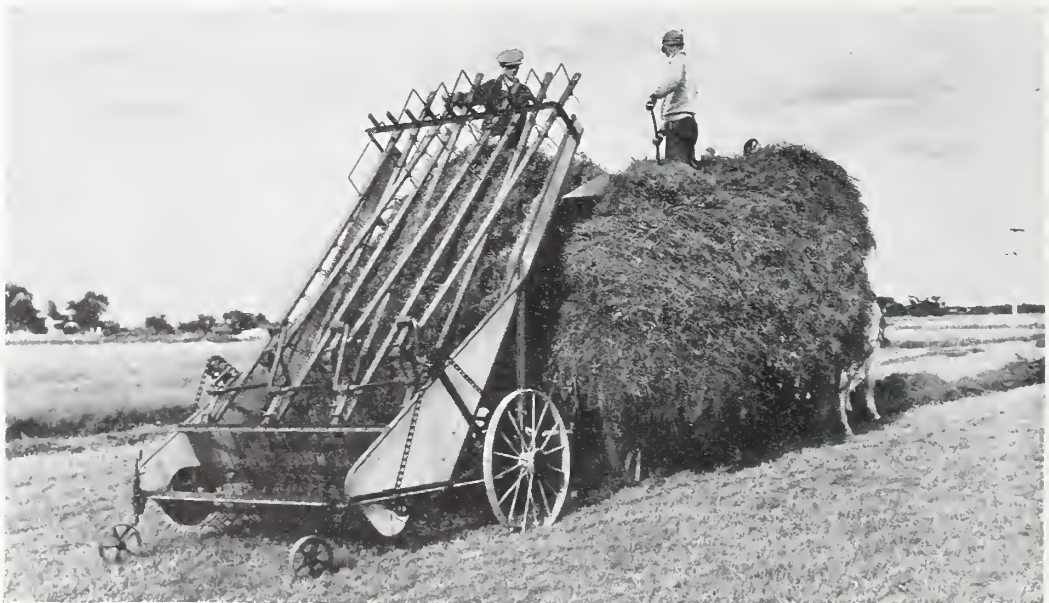
FIGURE 58.—Hay loaders are used principally in the Corn Belt and Northeastern States. When a hay loader is used for loading, and hay forks or slings are used for unloading, a crew of two men, one boy, and two horses can usually load, haul, and store about 10 tons of hay in 10 hours. When the hay is loaded and unloaded by hand the same crew could handle only about 5 tons in 10 hours.
