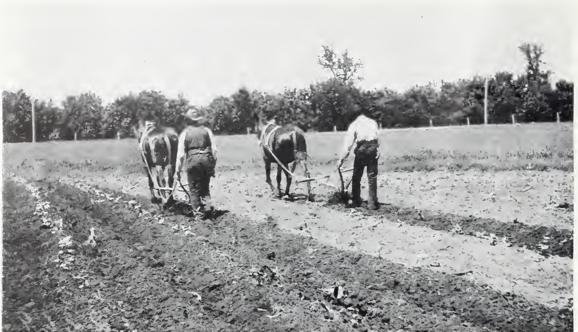
FIGURE 71.—One-animal cultivators are extensively used in the States of the old Cotton Belt, to the north, and along the Middle Atlantic seacoast. With cultivators of this type, two trips are needed to each row for every cultivation. Usually about 3 acres is a fair day's work for a crew of one man and one work animal when one-half-row cultivators are used.
