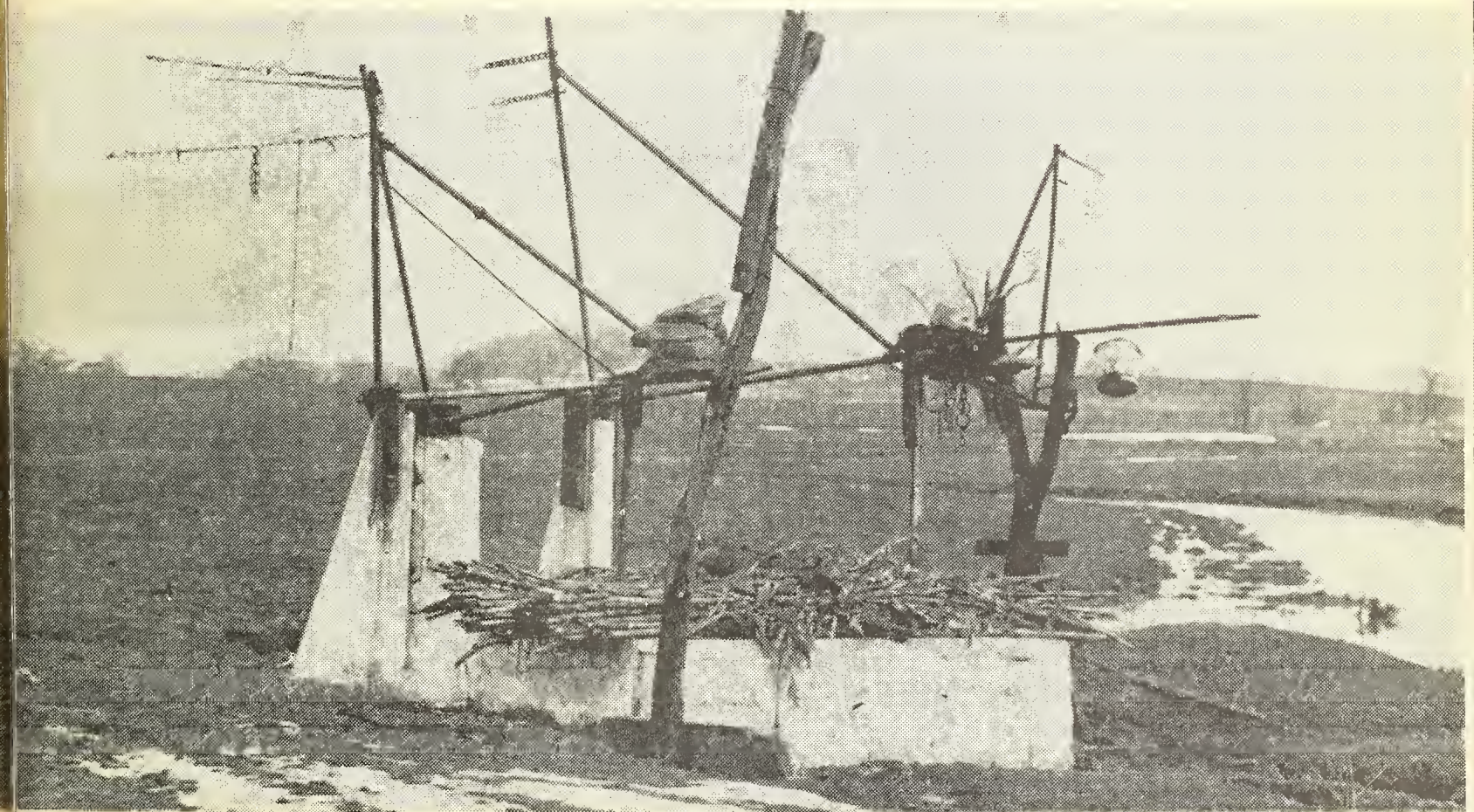
Figure 4.- The Old Order Amish and Old Order Mennonites living near streams still use water power to provide running water on the farm. In the concrete box is a water wheel which initiates alternating movements to the wires attached to the triangular-shaped devices. The movements of the wires operate short-stroke pumps located on 7 nearby farms, some 3/4 miles away. Water delivered by the pumps is circulated from the house
