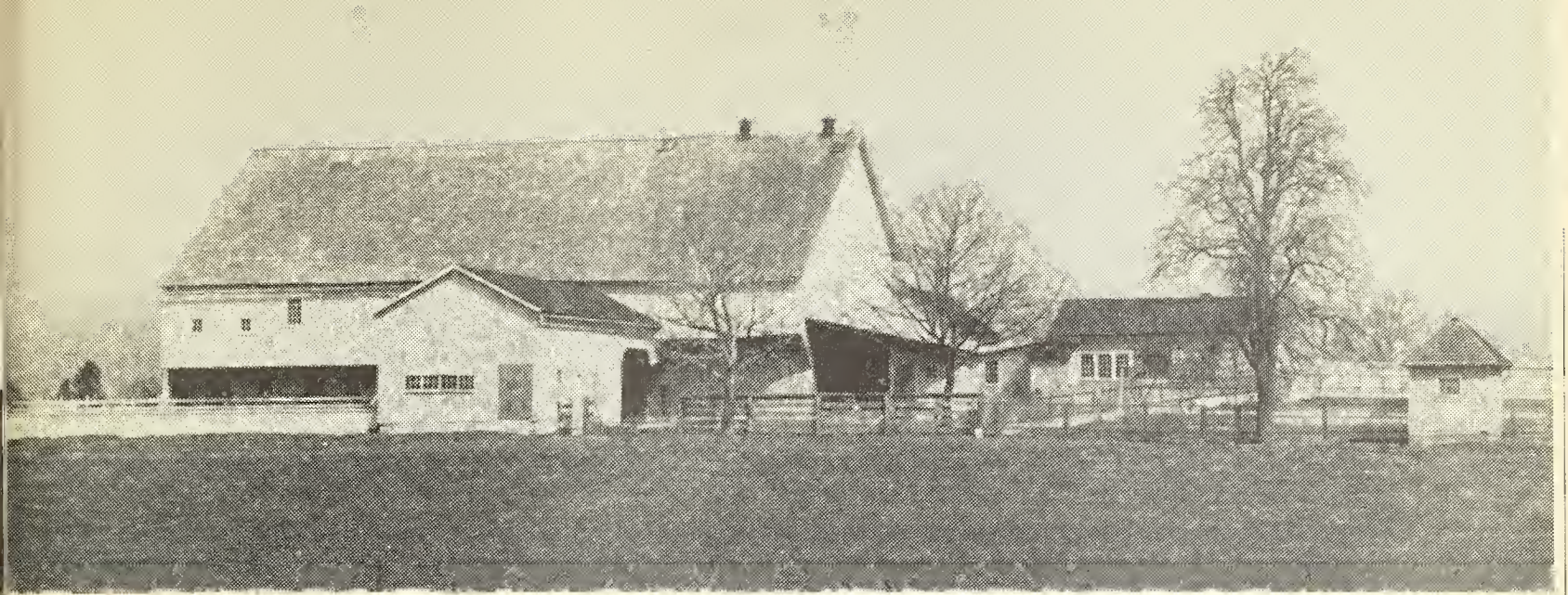
Figure 3.- The "overshot" (projection of the upper story over the lower) and the associated manure pen are retained in this Swiss or bank-barn.
