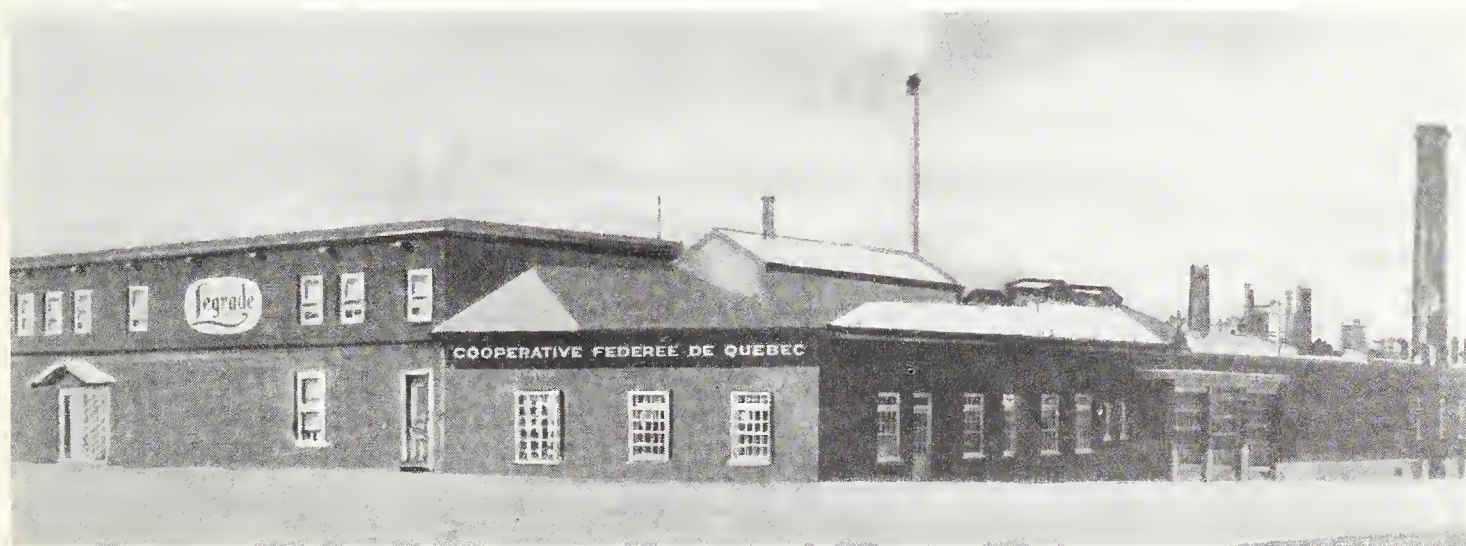
The Federee has operated this meat processing plant located at Princeville since 1922.
