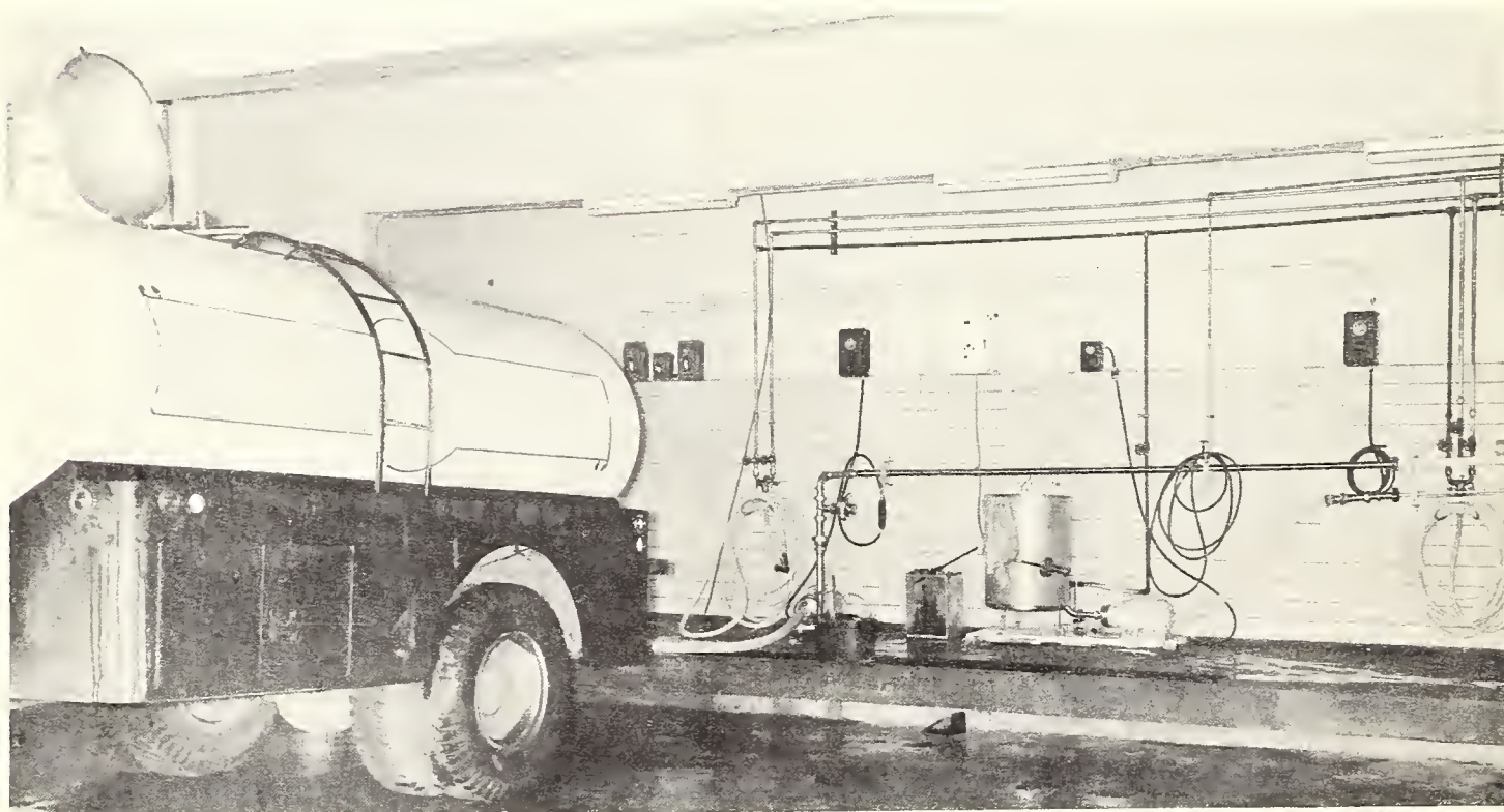
Milk receiving plants changing to an all-bulk operation have opportunities to reduce receiving costs significantly. This bulk receiving room illustrates the small investment in unloading equipment necessary for the bulk operation.
