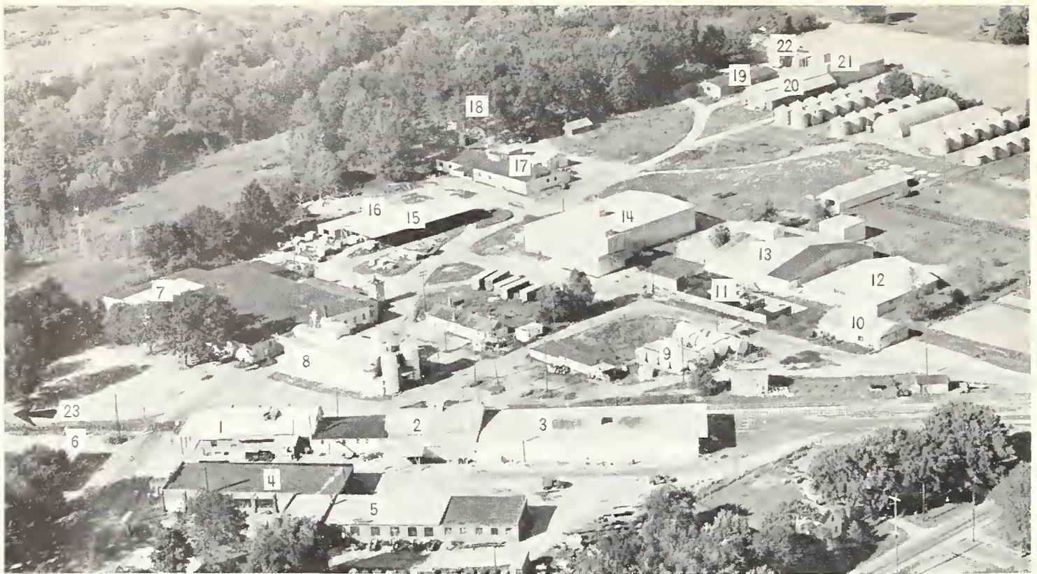
Aerial view of the Hamilton Farm Bureau Cooperative, Inc., Hamilton, Mich., with buildings identified: (1) Office; (2) old egg plant; (3) new egg plant addition; (4) garage; (5) implement; (6) hardware and appliances; (7) building supplies; (8) south feed plant; (9) oil plant; (10) oil truck garage; (11) coal yard; (12) warehouse; (13) fertilizer plant; (14) bulk feed ingredient plant and grain elevator; (15) lumber drying shed; (16) saw mill; (17) poultry processing plant; (18) and (19) implement warehouses; (20) ear corn drying crib; (21) ear corn elevator; (22) corn cob storage; and (23) north feed plant and bulk storage.
