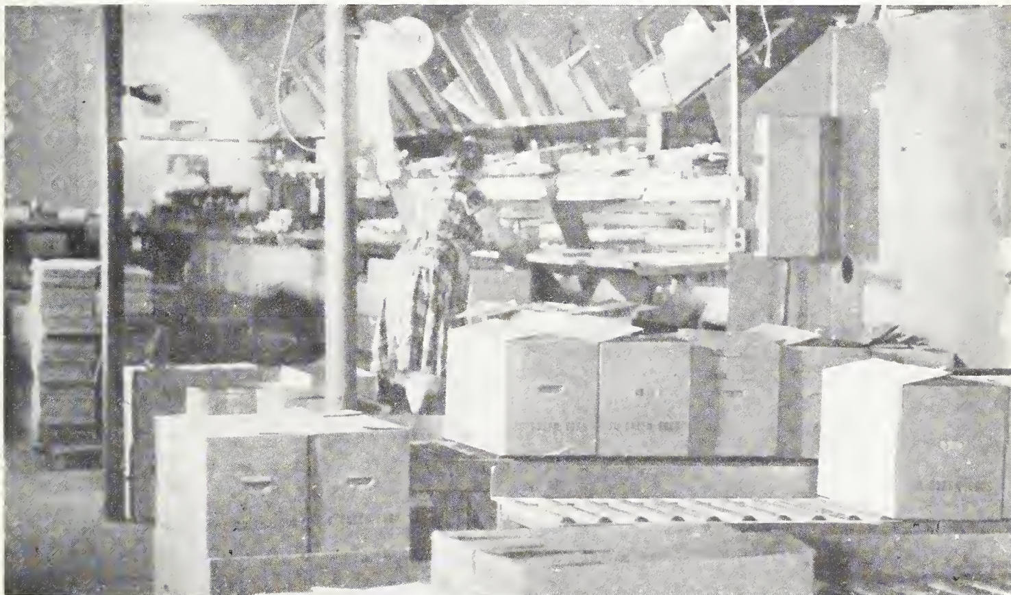
Electronic egg handling equipment installed by Hamilton Farm Bureau Cooperative to expedite the commercial egg enterprise of its members, the major operation of this co-op.
