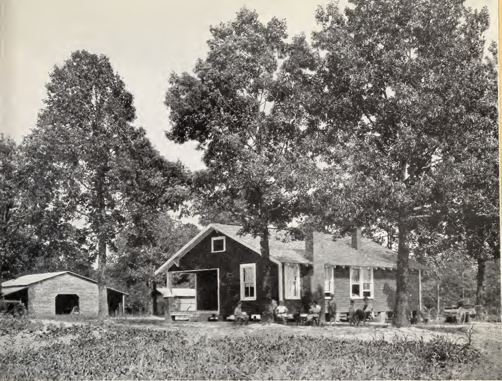
FIGURE 9.—Occasionally a tenant house is found that has real possibilities.
