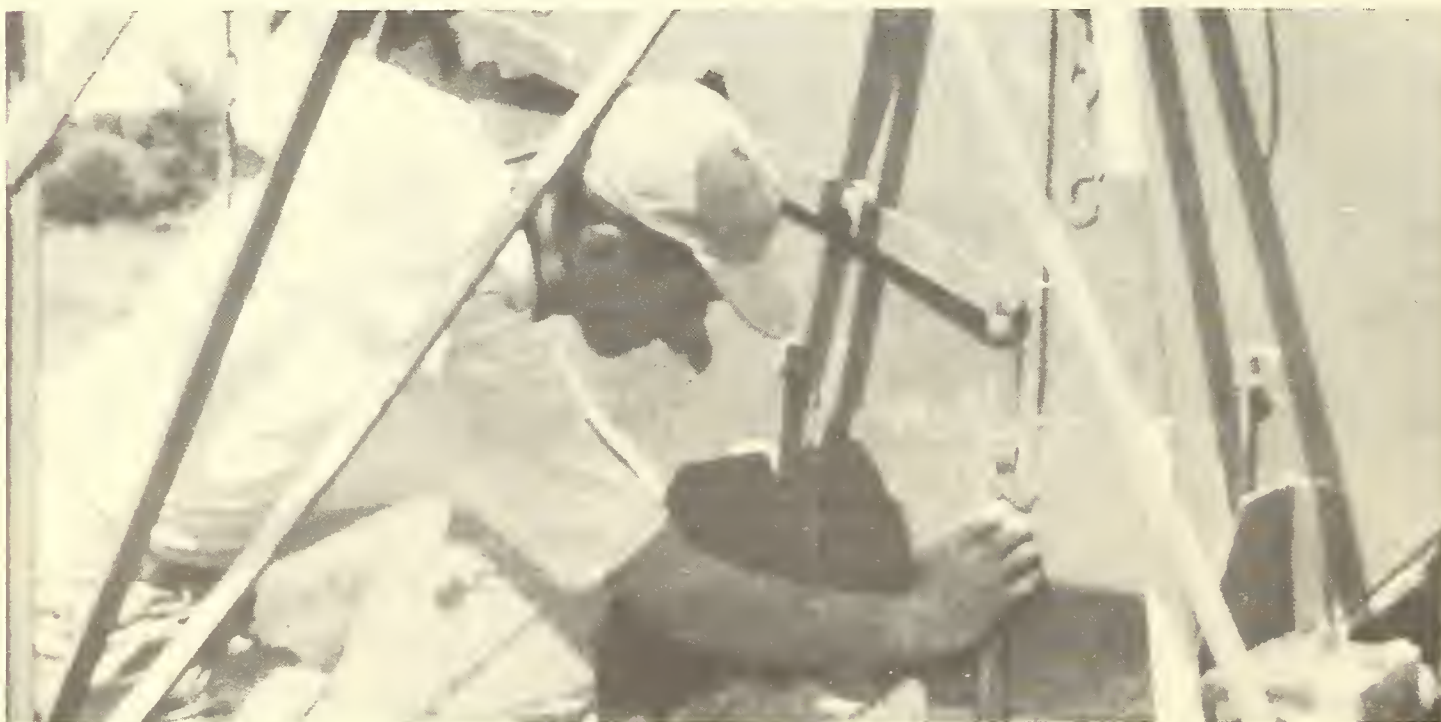
This operator is adjusting the rear gate of the spreader for proper application rate by means of a calibrated rule.
