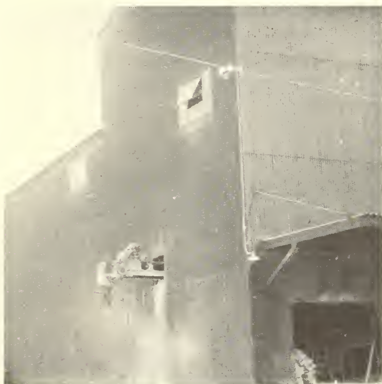
Loading chute on outside of plant is fed by belt conveyor leading from mixer. Fertilizer is weighed in payloaders before being dumped into bucket elevator that feeds mixer.
