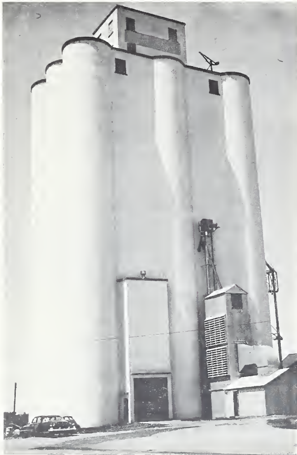
A modern country elevator, constructed of concrete, with grain drier installed as near the elevator as is workable. Insurance rates on this type elevator and drier are about one-fourth of those for a wooden elevator with drier. Most country elevators in Indiana lacked storage space necessary for drying.
