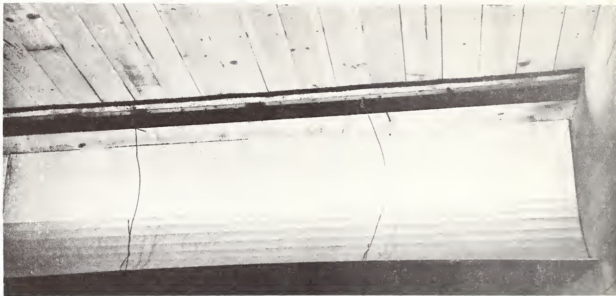
FIGURE 13.—View of air deflector inside a rectangular duct, directing air out through a slot in the top of the duct.
