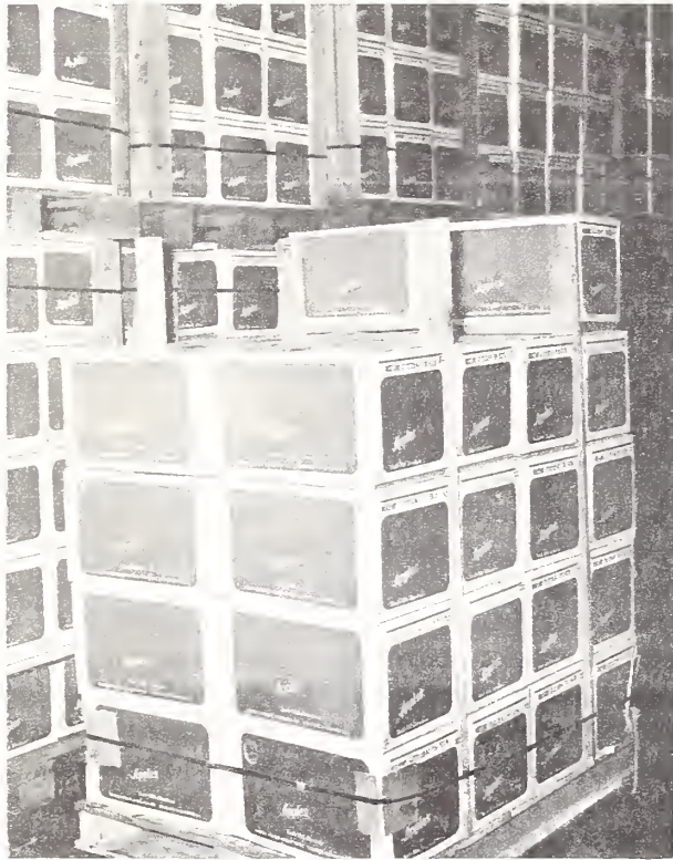
FIGURE 18.—Pallet load of fiberboard boxes of fruit spaced with 1- by 4-inch boards placed on end and other pallet loads with 1- by 4-inch corner boards to take load of pallet above.
