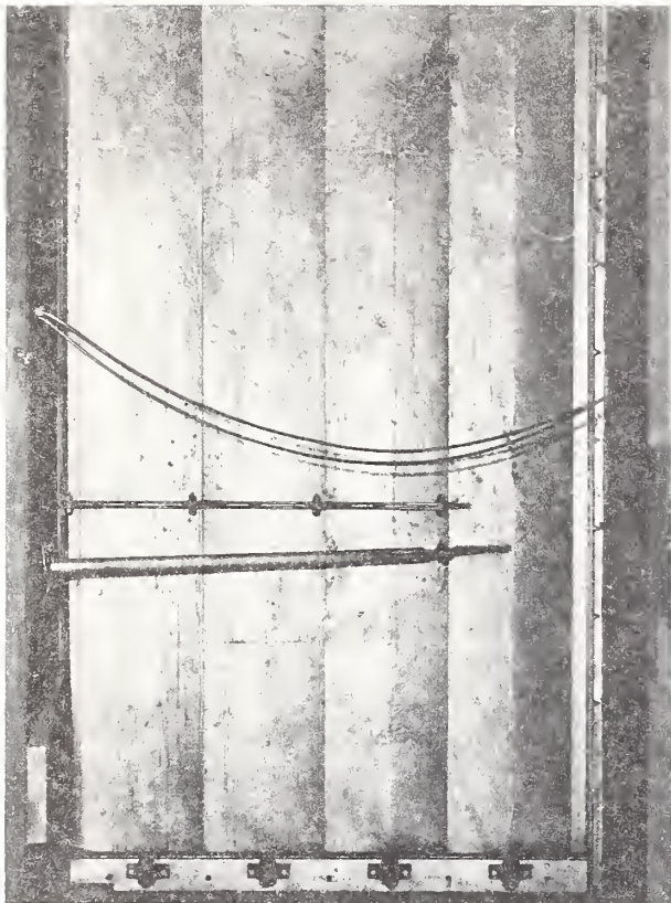
FIGURE 10.—Closed reversing dampers in a large air duct.
