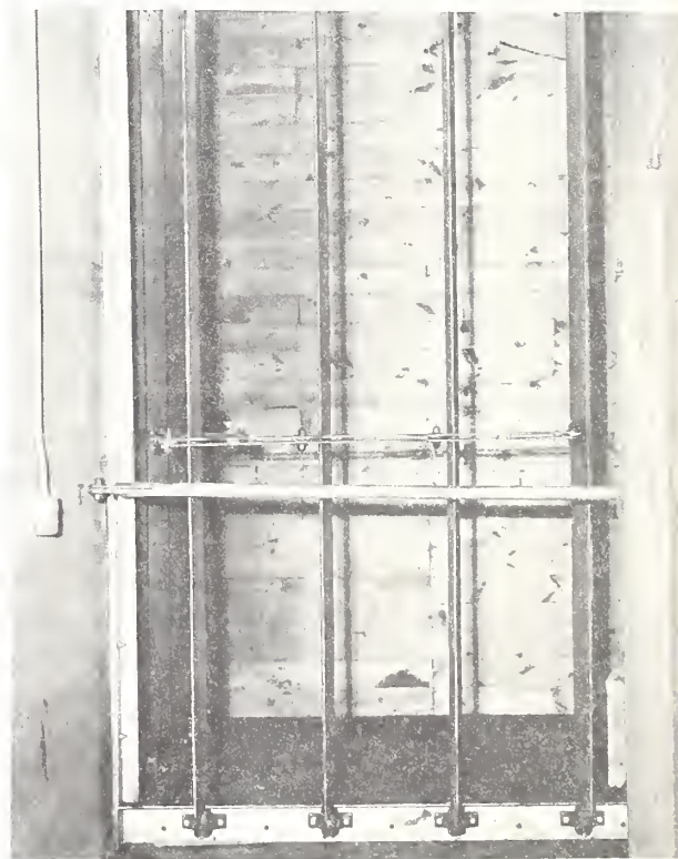
FIGURE 11.—Open reversing dampers in a large air duct.
