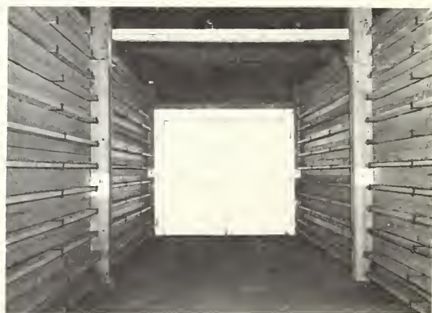
FIGURE 13.—Glued-tee type of bin front constructed at USDA Potato Research Center.
