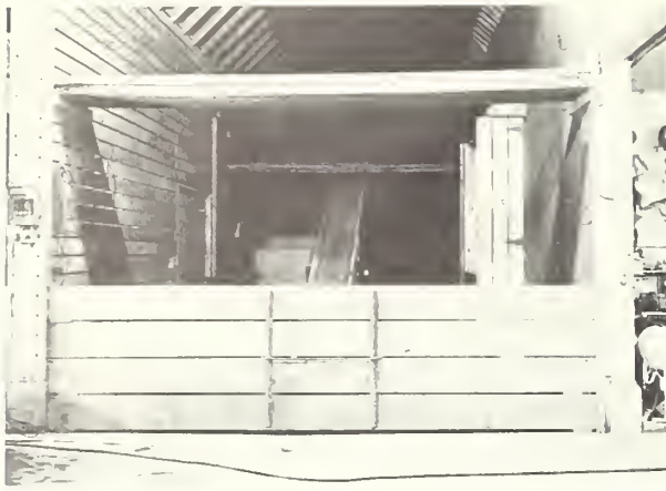
FIGURE 6.—Tie-back type of bin front strengthens straight panels spanning wide doorways.
