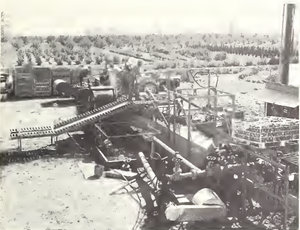
FIGURE 9.—Michigan State University (M.S.U.) pallet box dumper, flume, washing system as used in 1963.
