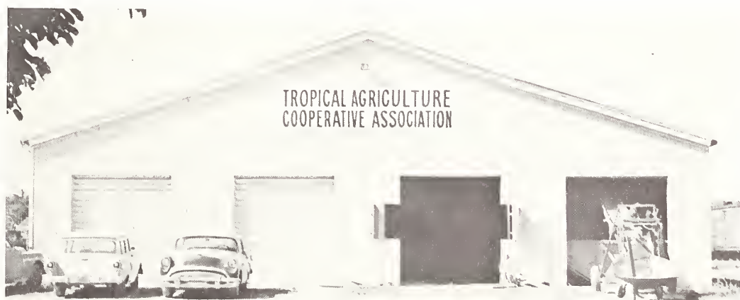
FIGURE 18.—Drive-in bin structure, front view. Each door opens into a bin approximately 100 feet long. A bin loader is in doorway of bin at right.
