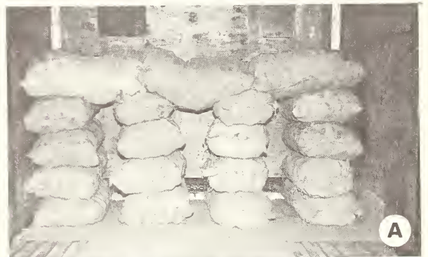
BN 23642, BN 23643 FIGURE 8. —Airflow pattern No. 4 for 100-pound burlap bags; for use in trailers with 2 inches of insulation or less. (A) First or header stack. (B) All subsequent stacks.
