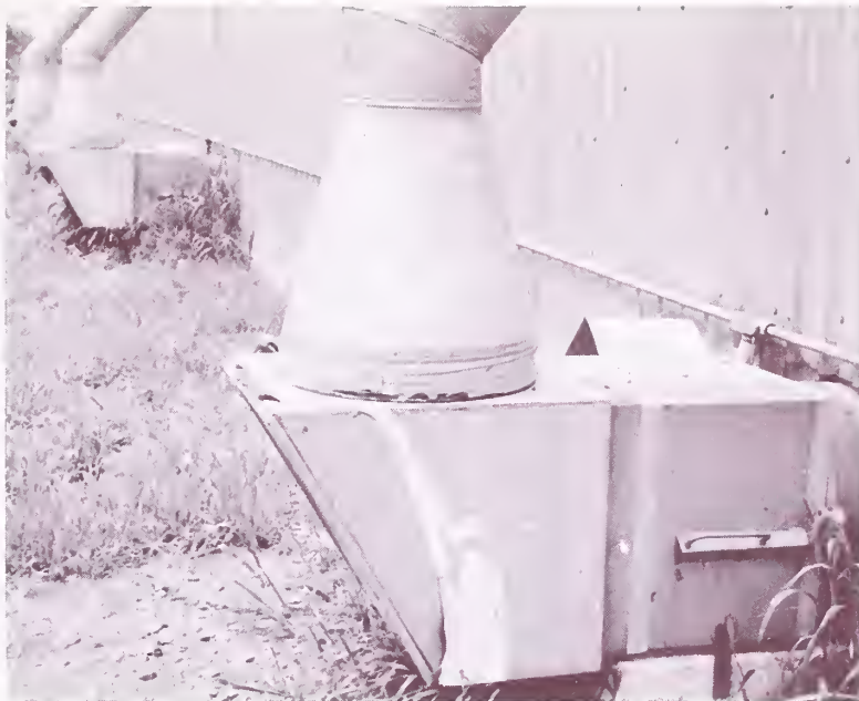
These three ducts are a part of the aeration system. Their purpose is to maintain the quality of the grain stored in this Kansas flat-storage facility.
