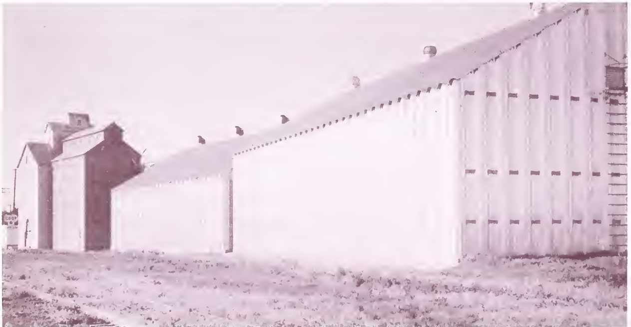
Most country elevators have expanded their storage capacity in recent years. These rectangular, flat, metal buildings (above) show the major form new expansion took.
