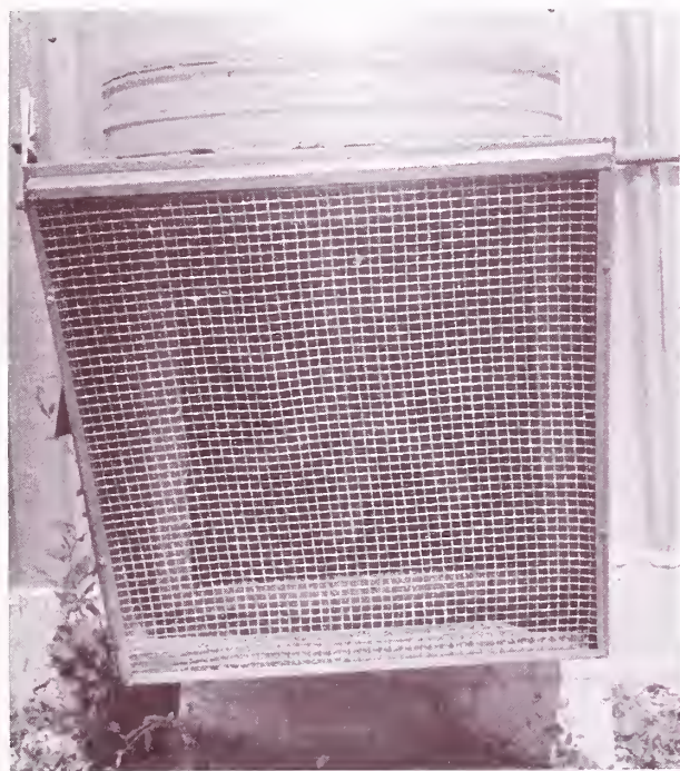
This "close-up" of an aeration duct indicates the relative size of the duct through which grain is aerated.
