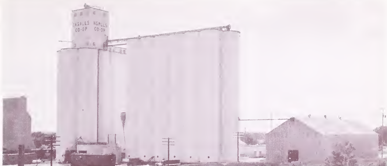
This concrete and flat building illustrates the way different types of storage structures are utilized in combination to satisfy the storage needs at many cooperative elevators.
