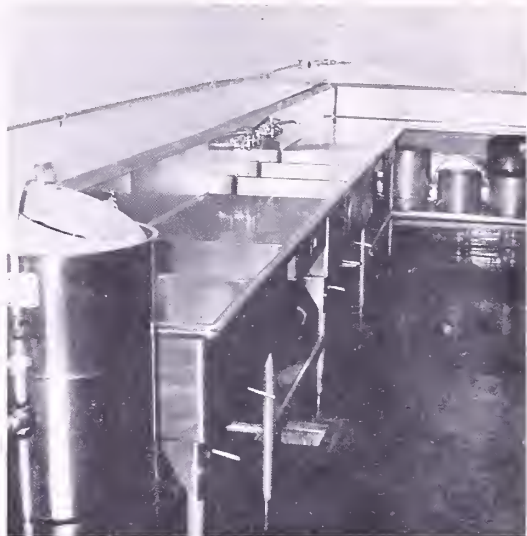
FIGURE 8.—Satisfactory arrangement of vegetable peeler, salad sink, and pot sink, with adequate drainboard space.
