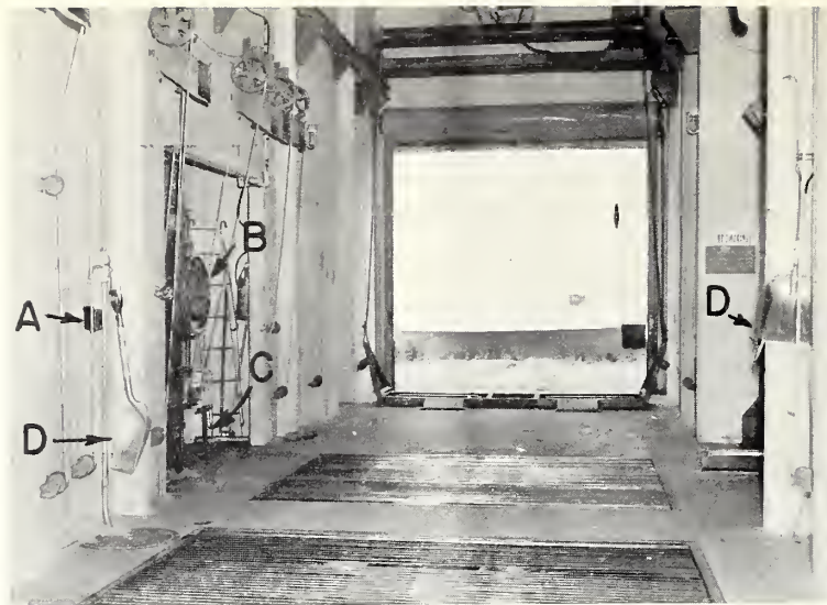
Figure 35. --Elevator driveway with two drive pits, viewed from entrance. Pit grating bars are placed crosswise of driveway. (A) The truck switch at the rear of the front pit. (B) The distributor wheel on the left side of the driveway near the pits. (C) Pit gate handle near drive pit. (D) Shovels located near rear of front pit.
