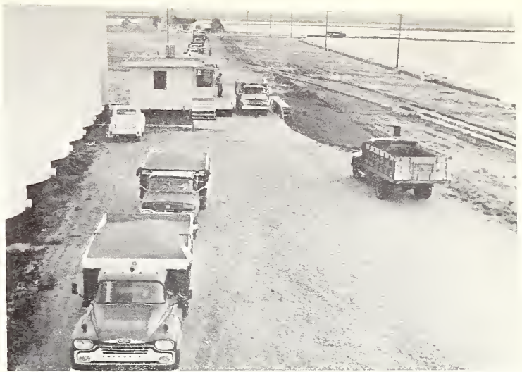
Figure 36.--Empty trucks cross the scale in the opposite direction of loaded trucks in conventional flow. Drivers of empty trucks are on the dock side of the scale. (Courtesy Hi Plains Journal, Dodge City, Kansas.)
