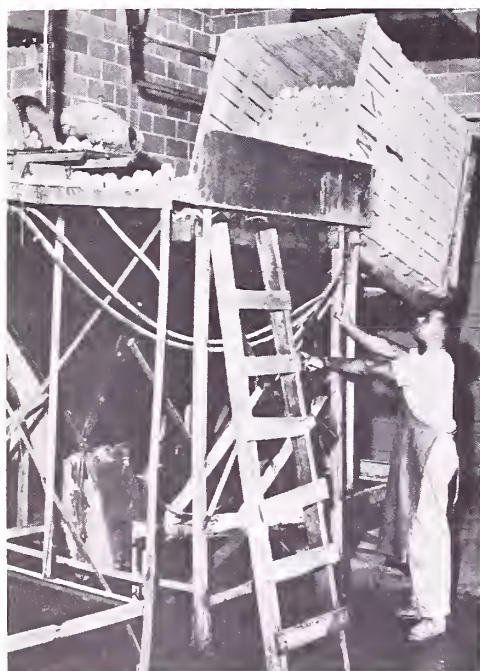
Figure 17.--Pallet box of potatoes is emptied by box tipper into the hopper that feeds the processing line.
