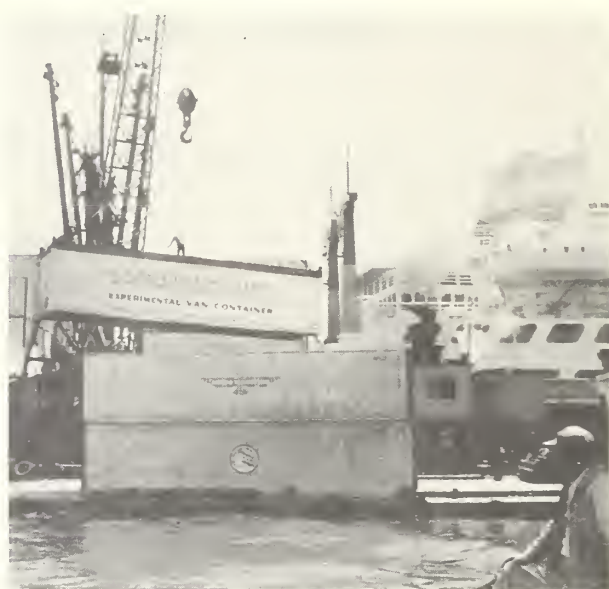
FIGURE 1.—USDA experimental van container being removed from ship at Pusan, South Korea.
