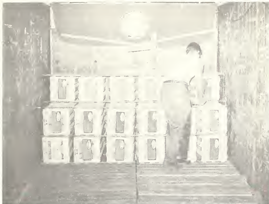
Figure 5.--The standard loading pattern and method of stripping conventional jumbo crates No. 1152 in a standard refrigerator car.
