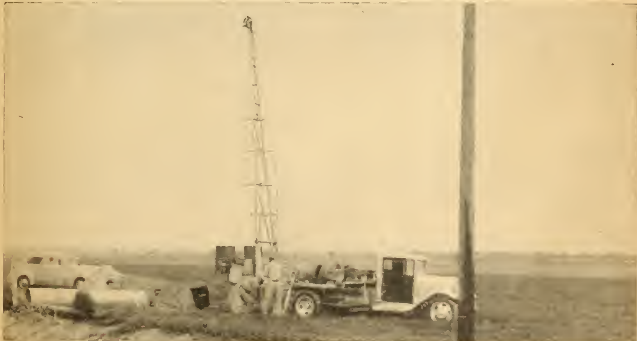
Drilling an irrigation well in the Republican Valley, Nebr.
