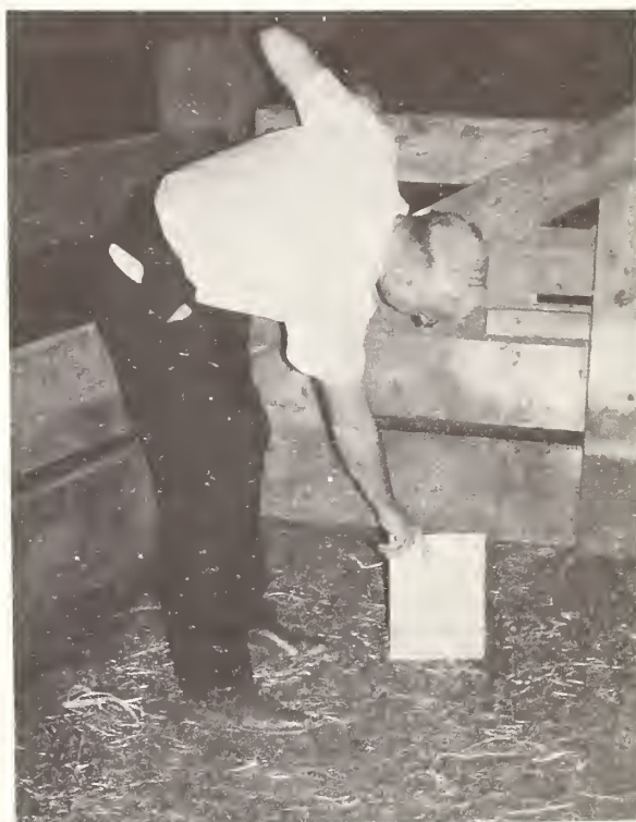
A 12-inch gap between the bottom of this gate and the floor is an invitation to disaster where small animals are concerned--especially when there is a steep, inclined rampway on one side as there is just beyond this gate. In the excitement of handling, the smaller animals often manage to get caught or wedged in the opening. Two hogs in one test slipped on the incline and were trapped under the gate. Both carcasses showed up in the cooler with severely bruised hams.
