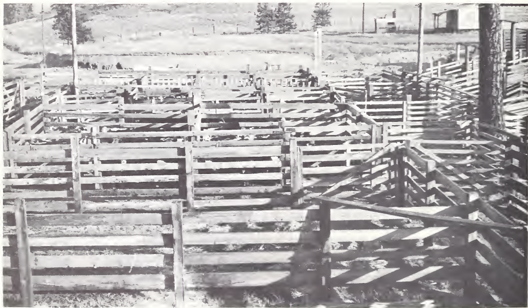
Holding pens of South Ferry Corral Association, Coleville Indian Reservation. Facilities were built in 1957 for a little over $3,000.
