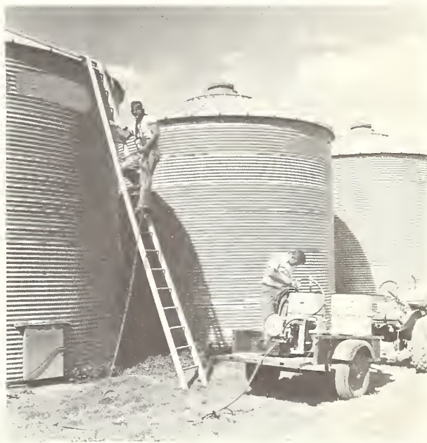
FIGURE 1—Pump and meter used to supply the liquid fumigants.
