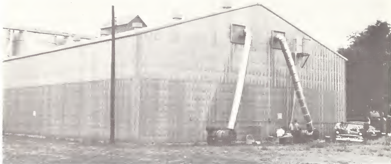
FIGURE 4.—Recirculation system in a Butler building at the Hart Grain Company, Woodston, Kans.
