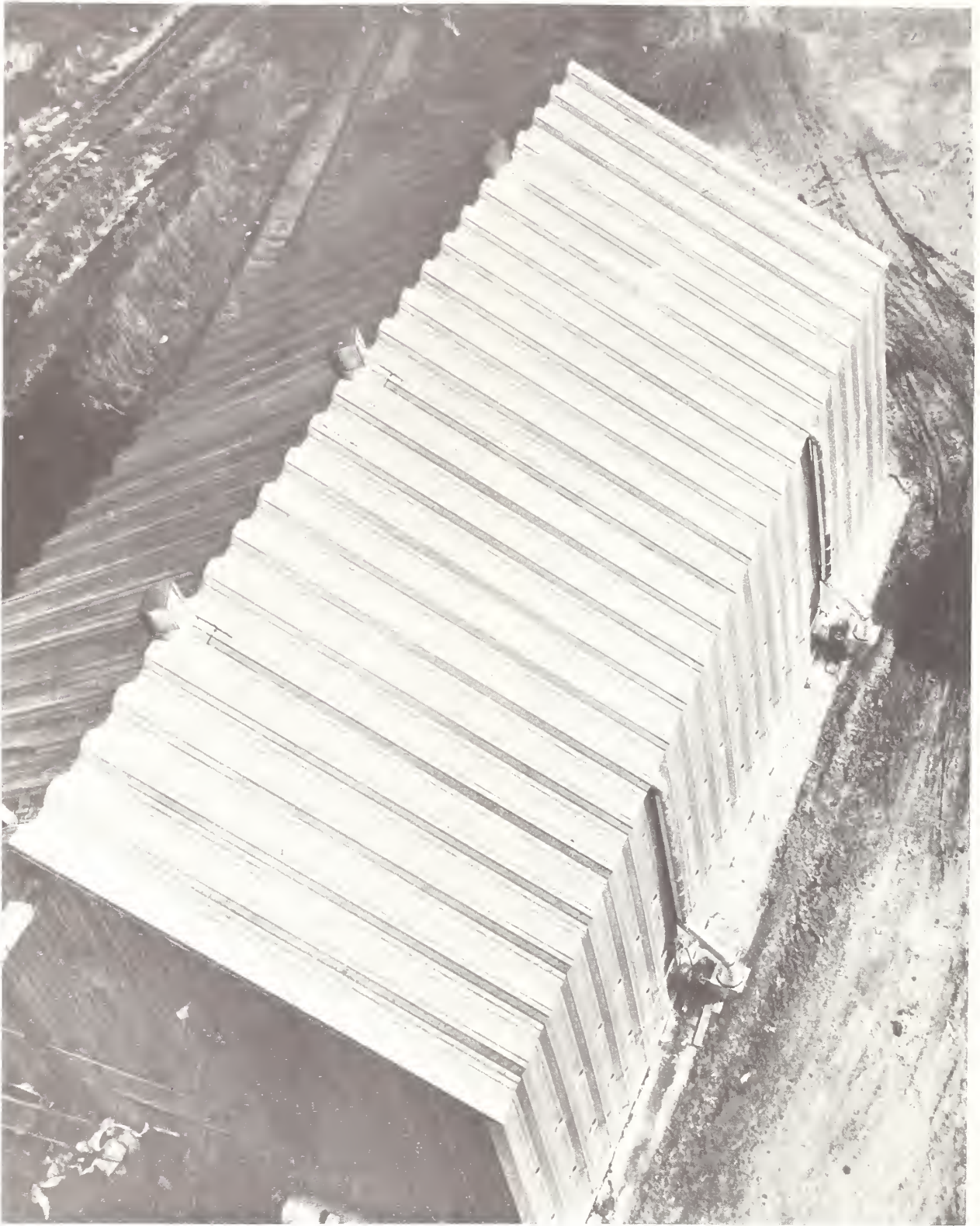
FIGURE 3.—Overhead view of Behlen building and recirculation system.
