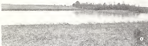
FIGURE 44.—Oxidation pond used for treatment of sewage and waste from a poultry-processing plant.
